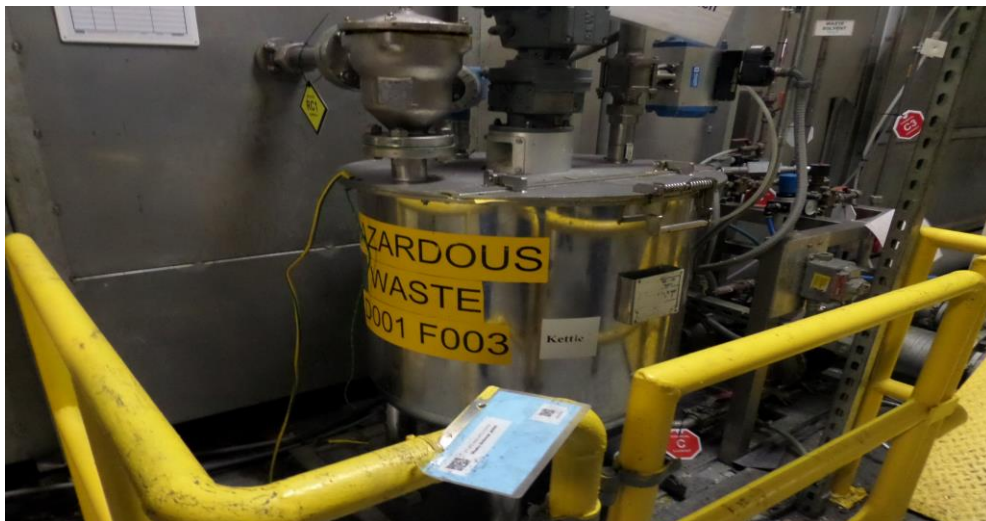
Hyundai. Kettle Purge Tank 2 Area. Inspectors observed a 35-gallon purge tank (tank 2) accumulating waste paint and solvent. The inspectors observed the tank was not marked/labeled with an indication of the hazards. Inspectors observed red octagonal shaped lockout tags and yellow diamond shaped tags designated with the letters C, P, E or RC and followed by a number (1, 2, or 3) secured by plastic cable ties to the tanks and the tank's ancillary equipment (valves, pumps, flanges, connectors, electrical and pneumatic equipment). Photograph 12 taken July 26, 2021 at 3:50 p.m.
