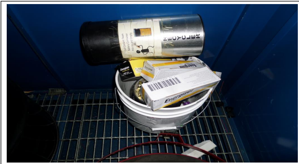
Hyundai. Engine Building 2 90-Day Area. Inspectors observed a 5-gallon container accumulating waste batteries in a metal storage locker with secondary containment. The inspectors observed the container was not marked/labeled with the words universal waste and not marked with a date. The facility corrected the deficiency by labeling the container with the words universal waste. Photograph 24 taken July 27, 2021 at 11:30 a.m.
