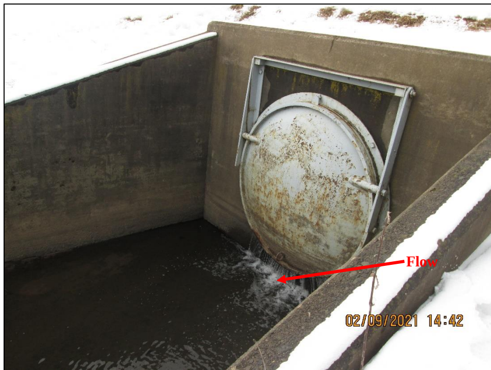
Photograph 44. View, facing west, of the pipe flap gate for Outfall WB18. Flow was observed from the outfall. City representatives stated that an unnamed creek contributes to this outfall, so flow is expected.
