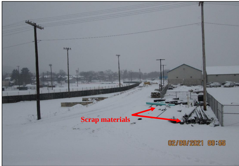
Photograph 6. View, facing east, of stockpiled materials stored uncovered along the northwestern edge of the Municipal Complex property.
