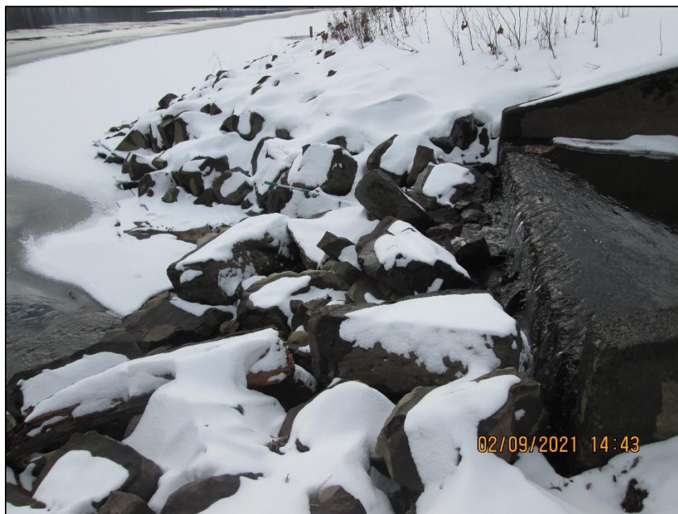
Photograph 45. View, facing southwest, of rip rap at the end of the Outfall WB18 headwall.
