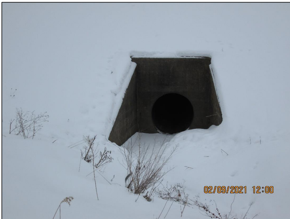
Photograph 29. View, facing south, of the headwall at the southwest corner of the Grey Fox Rentals SMP. This headwall is on the north side of a large levee and Outfall DR01 is on the south side of the levee.
