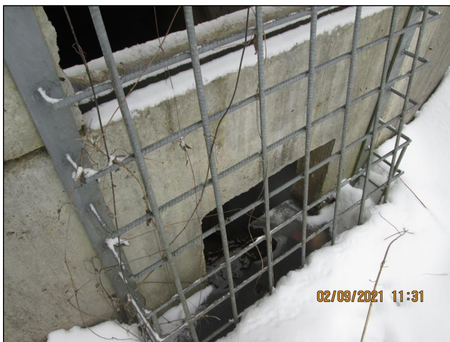
Photograph 25. Closer view of trash rack located near the BMP's outlet.
