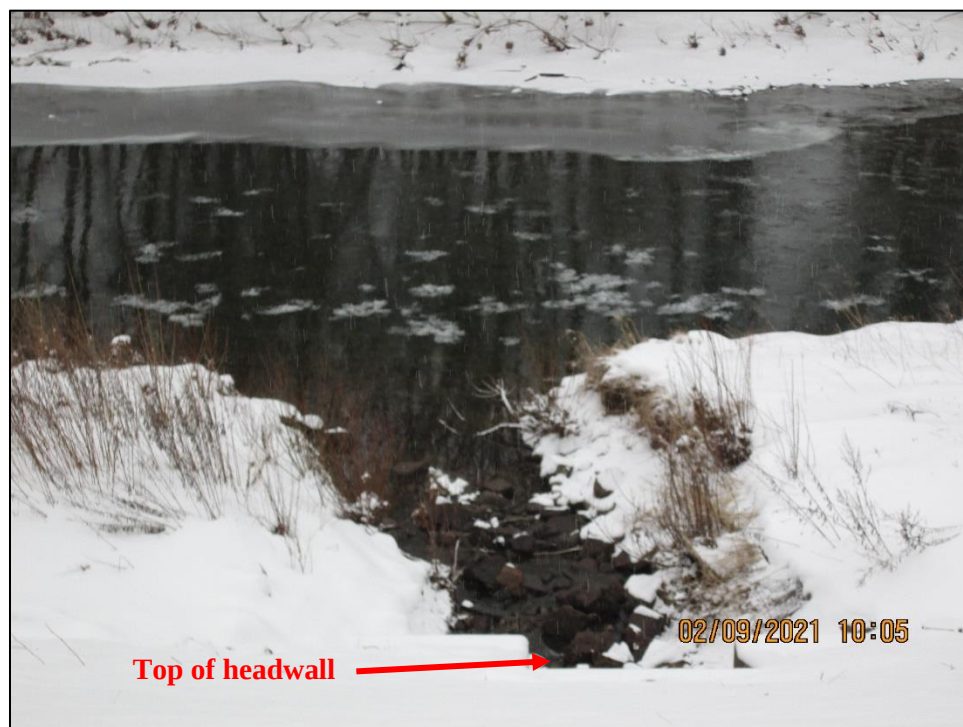
Photograph 21. Zoomed-in view, facing west, of Outfall LY06. The top of the headwall and the short channel between the outfall and Lycoming Creek are visible.
