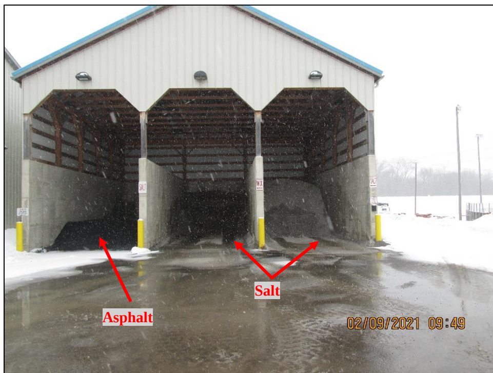
Photograph 4. View, facing west, of one covered asphalt bin and two covered salt bins along the western boundary of the Municipal Complex.
