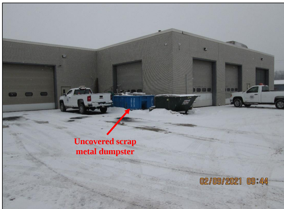
Photograph 2. View, facing southeast, of an uncovered scrap metal dumpster outside of the Public Works building.
