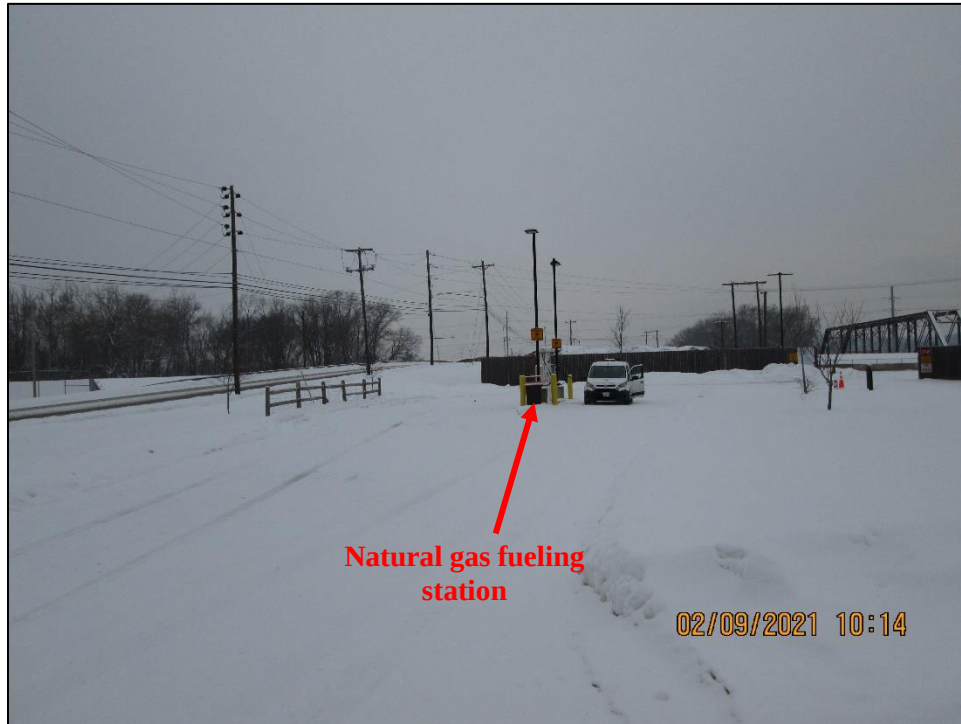
Photograph 8. View, facing west, of a public access compressed natural gas fueling station located near the southwest corner of the Municipal Complex.
