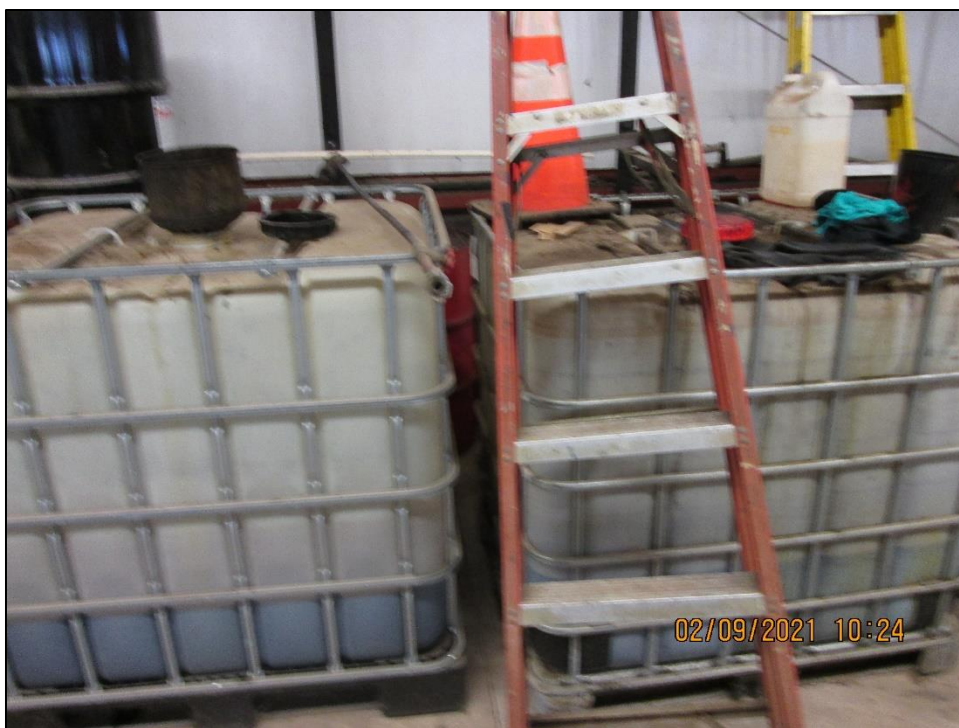
Photograph 11. View of two partially filled 330-gallon totes containing used oil inside of the “American Building.” All containers were inside of a covered building, but lacked secondary containment.
