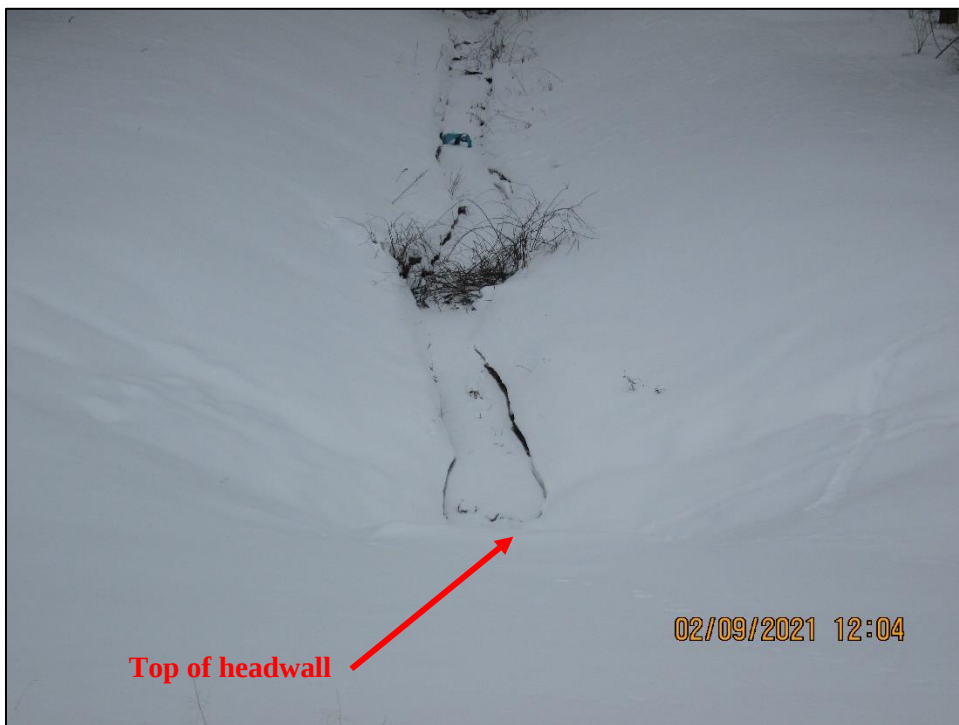
Photograph 30. View, facing south, of the top of the headwall for Outfall DR01. No flow was observed in the unnamed ditch running to the south from the outfall.
