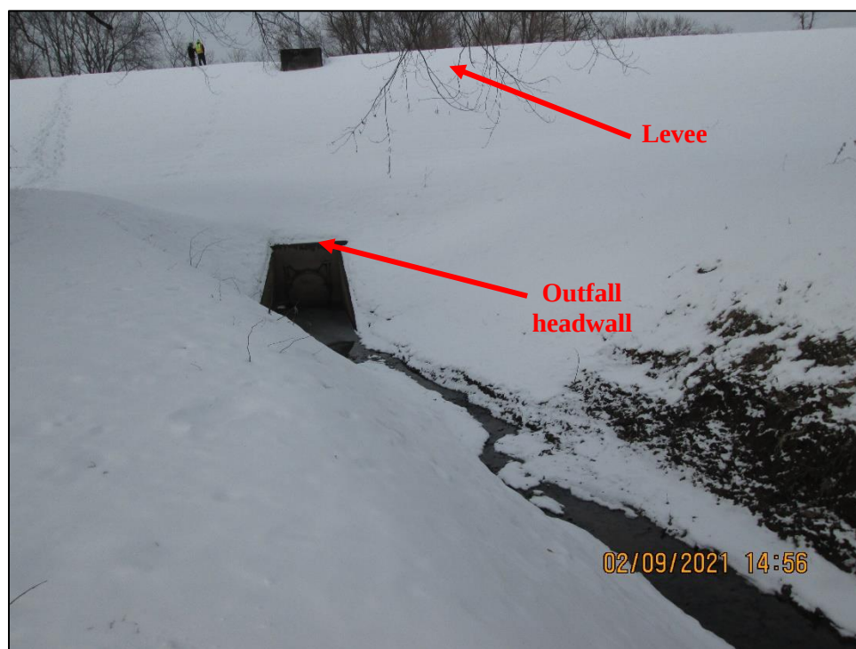
Photograph 46. View, facing northwest, of Outfall WB19 at the base of a levee. This outfall flows to a small ditch running to the West Branch Susquehanna River.
