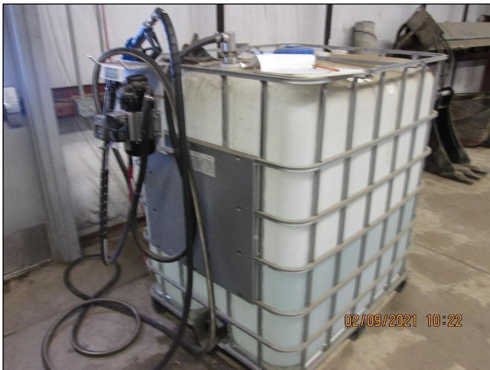
Photograph 12. View of one partially filled 330-gallon tote containing diesel exhaust fluid inside of the “American Building.” All containers were inside of a covered building, but lacked secondary containment.
