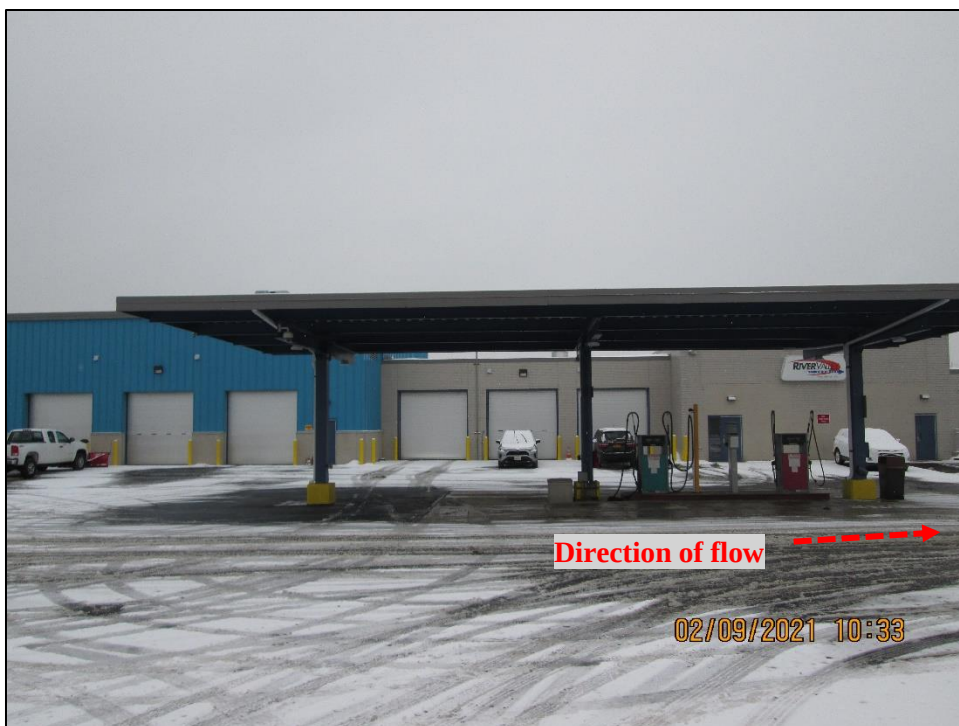
Photograph 15. View, facing east, of a covered bus fueling station for gasoline and diesel. A spill kit was present. Spills from this area would appear to flow downhill southward to a storm drain in the employee parking lot of the River Valley Transit building.
