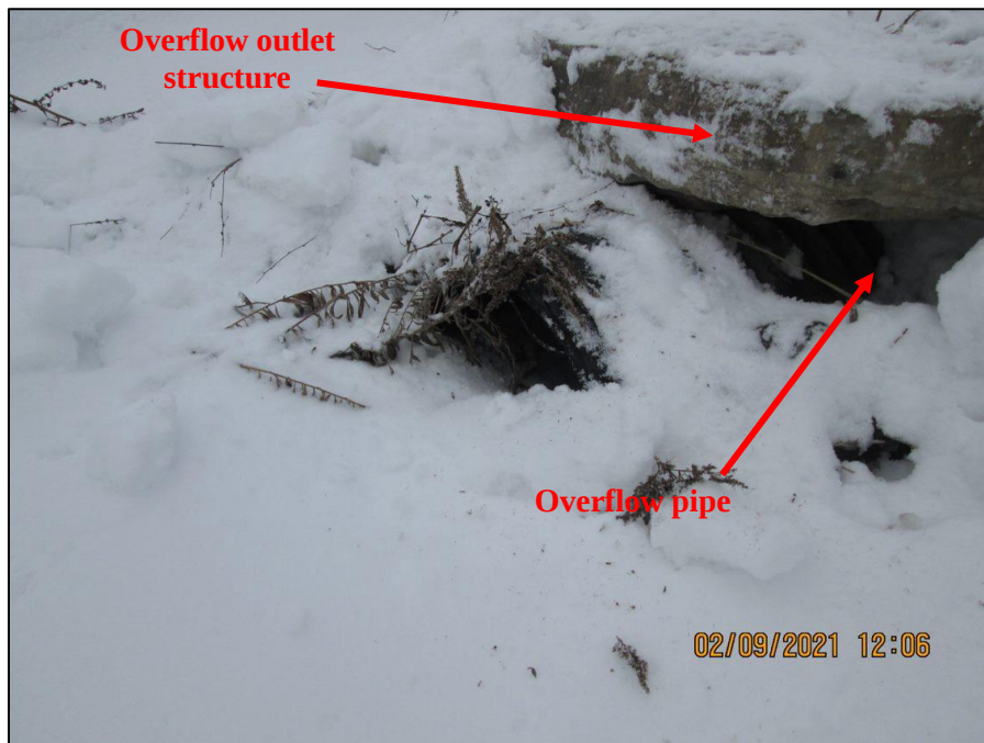
Photograph 28. View facing northeast, of the overflow structure for the SMP. Though not observed during the inspection, drainage from the SMP would flow into a drainage ditch and south towards Daugherty Run.
