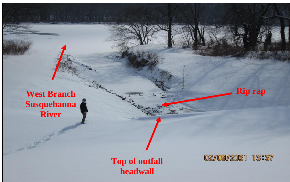
Photograph 38. View, facing south, of the top of the headwall for Outfall WB01. Rip rap was observed in the ditch between the outfall and the West Branch Susquehanna River.
