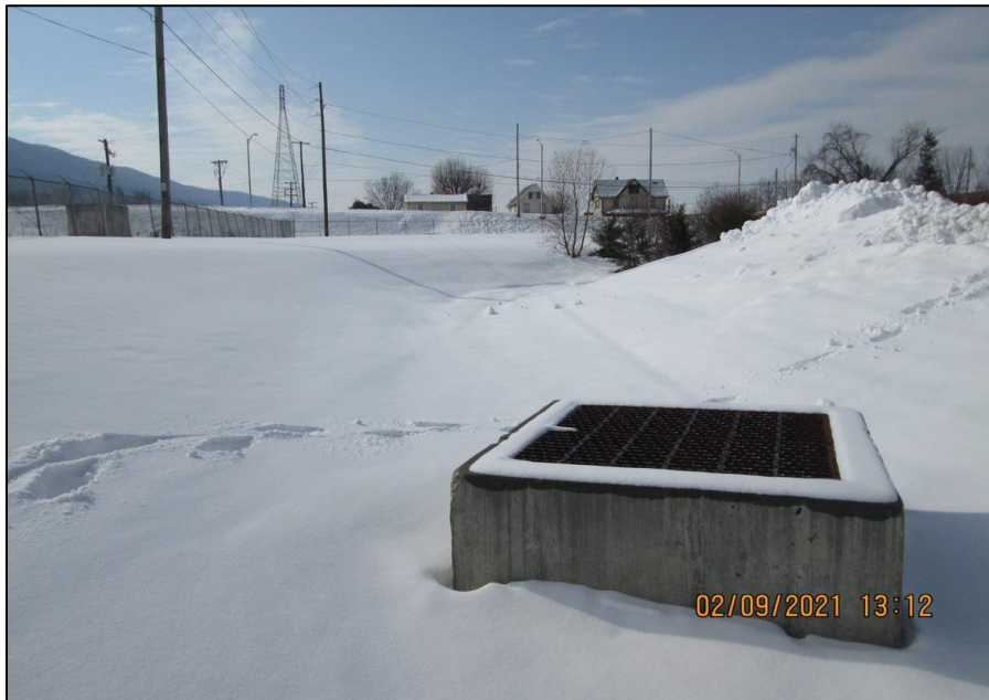
Photograph 36. View, facing southwest, of the concrete riser structure located in the middle of the vegetated swale. The riser contains the 30-inch stormwater pipe that conveys stormwater through the levee and into the Susquehanna River.
