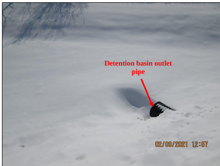
Photograph 33. View of the outlet inside the detention basin. Note the detention basin receives sheet flow coming from the adjacent parking lot.
