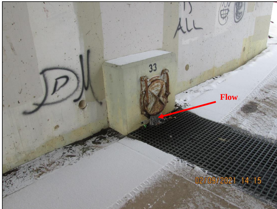
Photograph 40. View, facing northeast, of Outfall WB10. Flow was observed at the bottom of a pipe flap gate.
