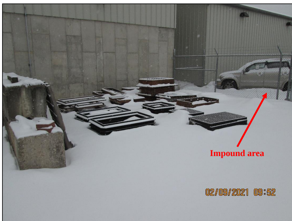
Photograph 5. View, facing southeast, of the uncovered stockpiled materials and the uncovered vehicle impound area. The City foreman stated that the impound belongs to the police, but stated that they did not know if vehicle fluids were emptied before vehicles were stored.
