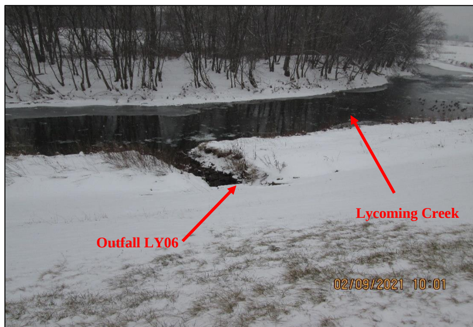
Photograph 20. View, facing west, of Outfall LY06 to Lycoming Creek. Flow was observed from the outfall.
