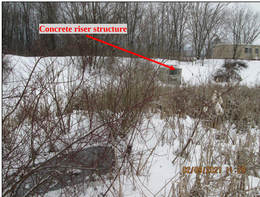
Photograph 23. Closer view of the detention basin from Photograph 22. Note the concrete riser structure with trash rack.
