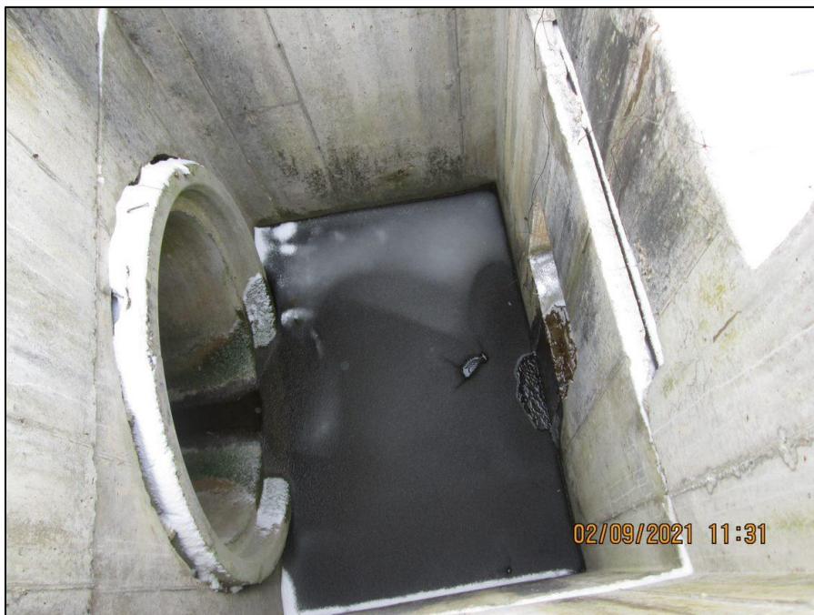
Photograph 26. View inside the concrete riser outlet structure. It should be noted there was no observable trash at the time of the inspection.
