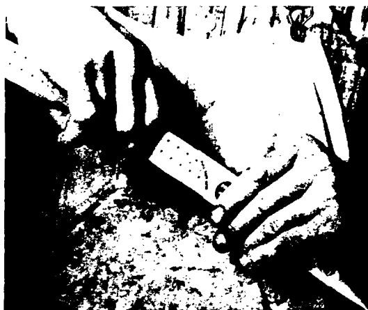
23. FOLDING PERF-A-TAPE— The Corner Fold, included with each package, is wrapped around the tape, which is then pulled through, quickly creasing the Perf-A-Tape in the center.
