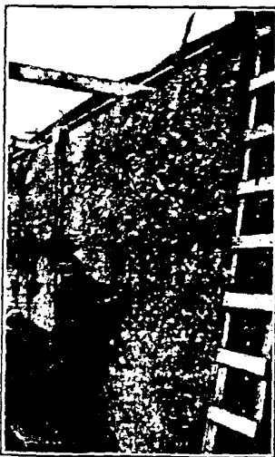
Three steps in re-facing Montreal docks. AT LEFT, inserting nails secured by lead expansion bolts in concrete; CENTER, spraying gunitite over steel mesh held by nails; RIGHT, the new finished surface.
