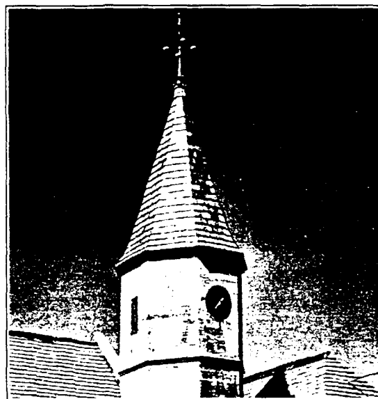
Lead clock face on the library tower. Lead flashing is visible along sloping coping.
