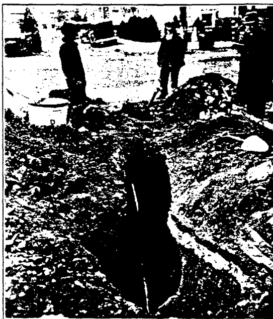
Installing a 2 in. lead water service at a busy Long Island corner. Note flexibility of the pipe.
