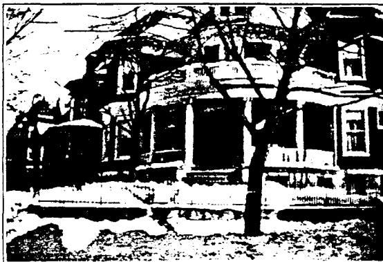
White lead painted trim on a home in the Bronx, New York City. Painted 1928 and 1934.
