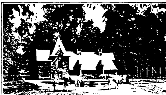
Stables on the Kean estate. The ventilators in the roof are flashed with lead.
