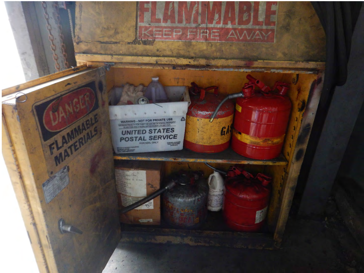
# 241 – Flammable Materials Cabinet
