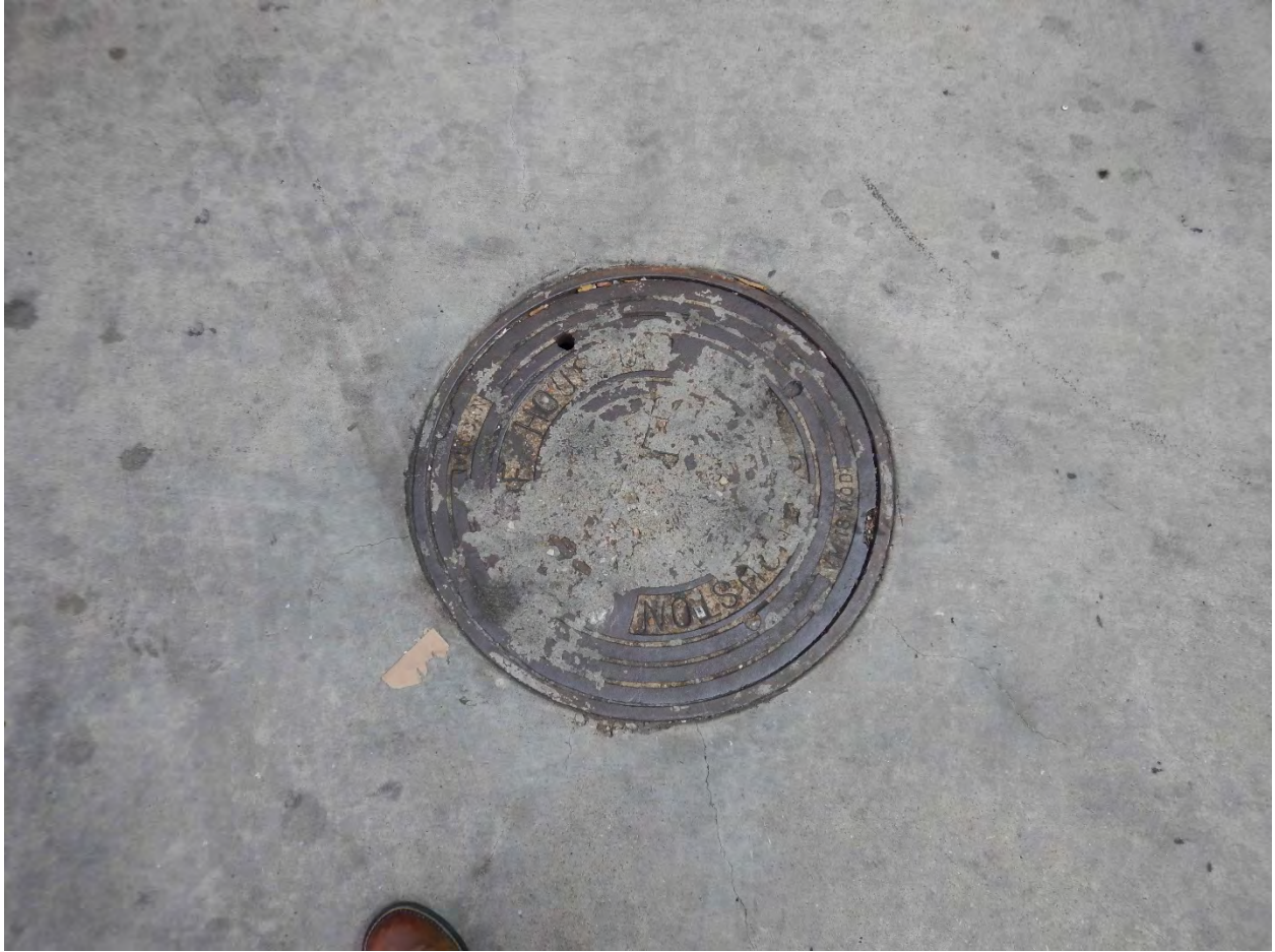
# 253 – Underground Storage Tank Cover
