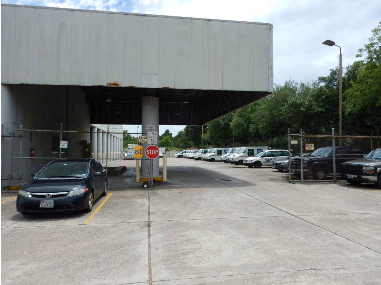
# 284 – Vehicle Entrance of Facility
