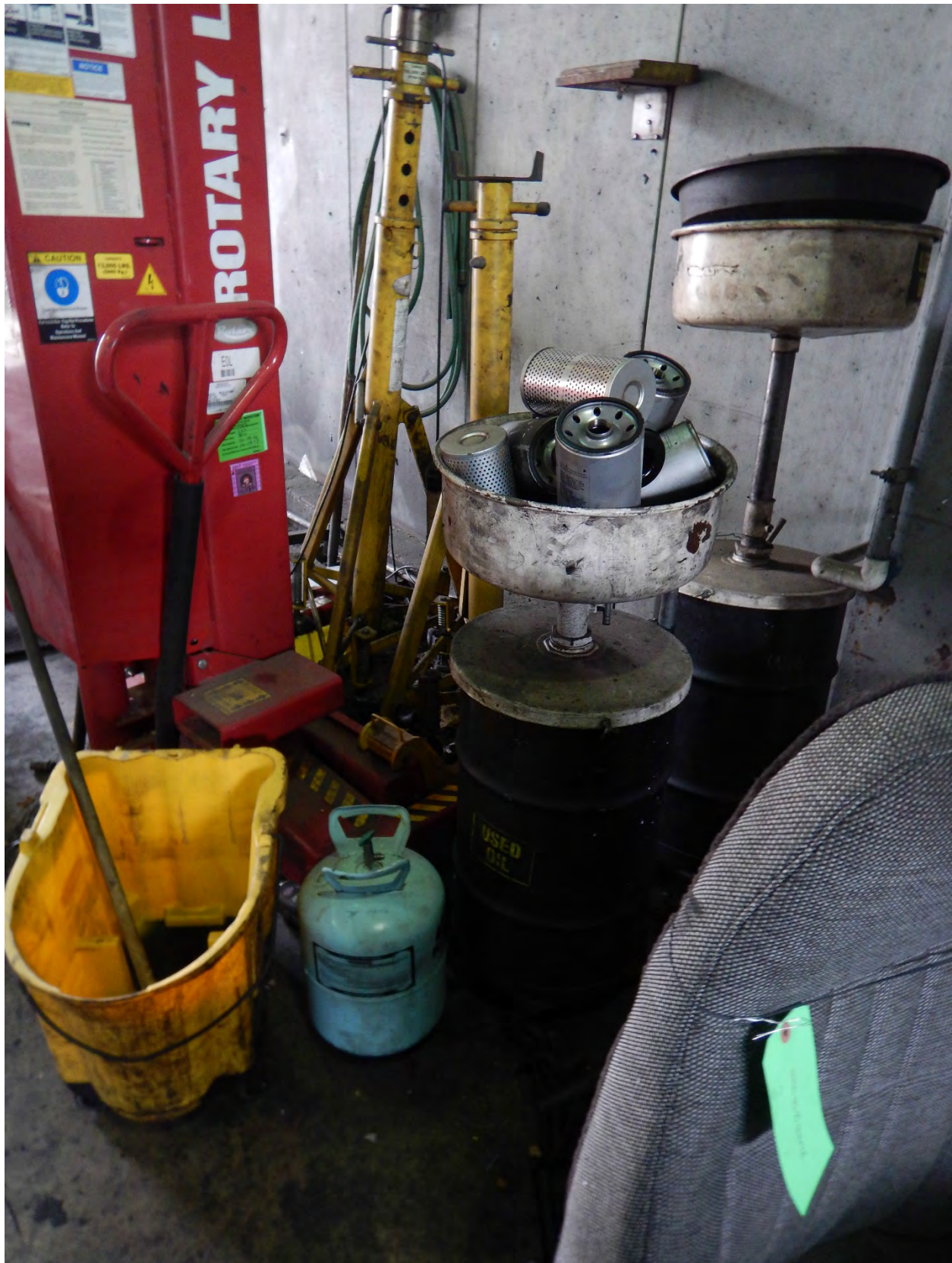
# 235 – Filter/ used oil drain Area # 5
