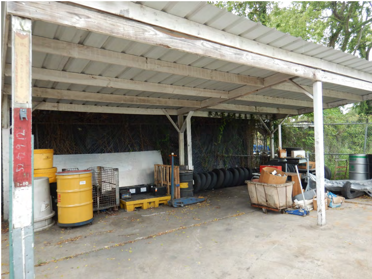
# 256 – Wide shot of outside storage area
