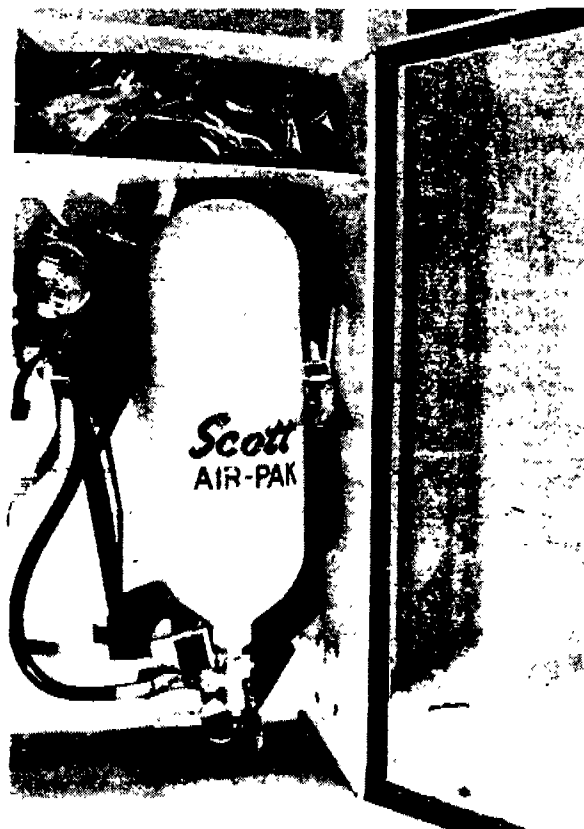
Figure 9-6. Wall-mounted storage cabinet for a SCBA.
