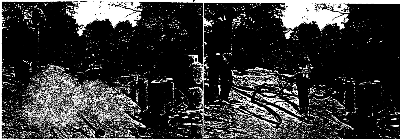
Figure 13. Dust from rock drilling operations, uncontrolled and controlled by dust trap.
