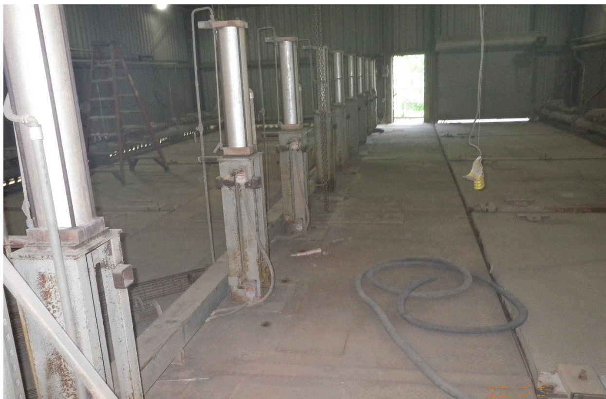
11. Top of Boiler 2 Baghouse (not operating) – Panther Creek Generating – 6/8/22
