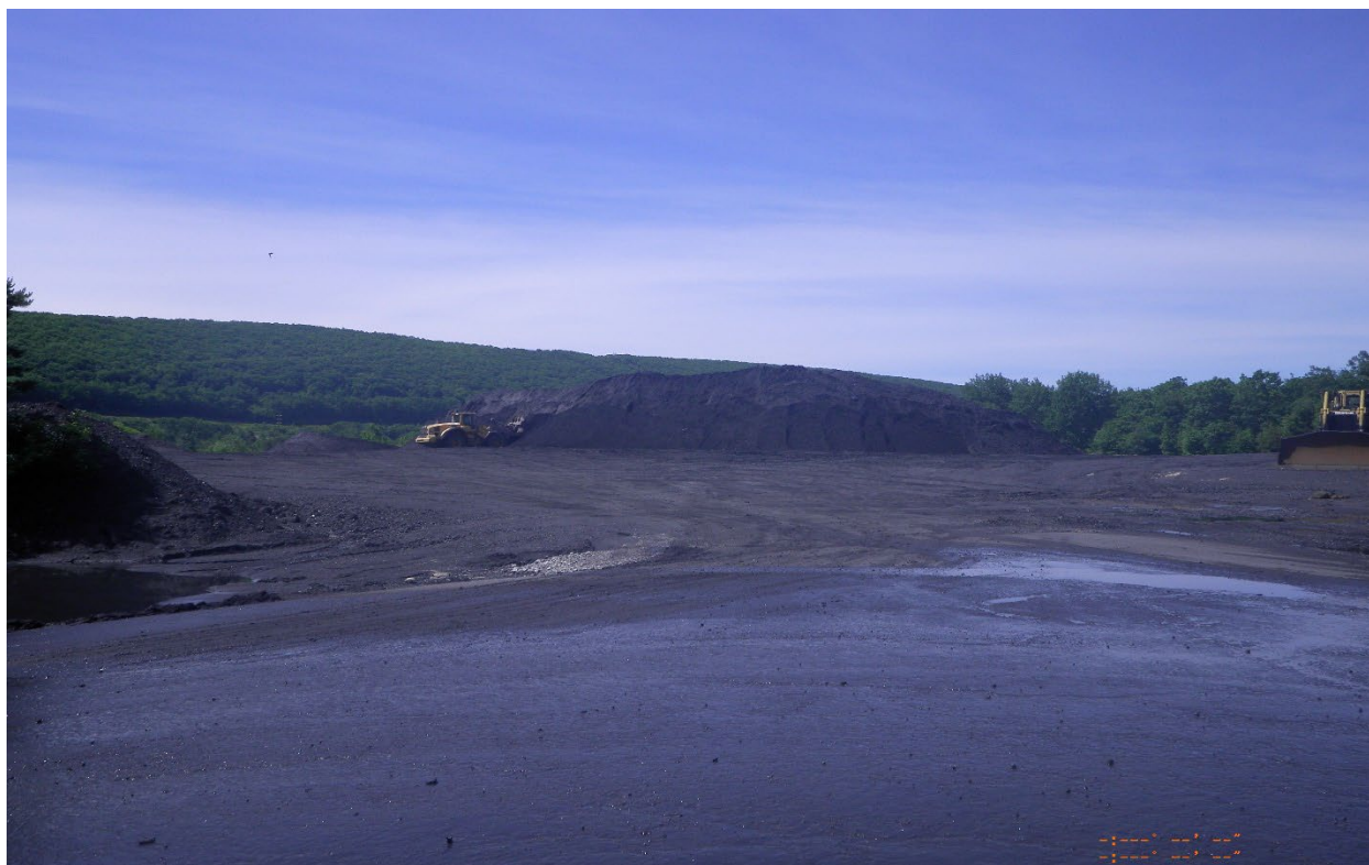
1. Waste Coal Pile – Panther Creek Generating – 6/8/22
