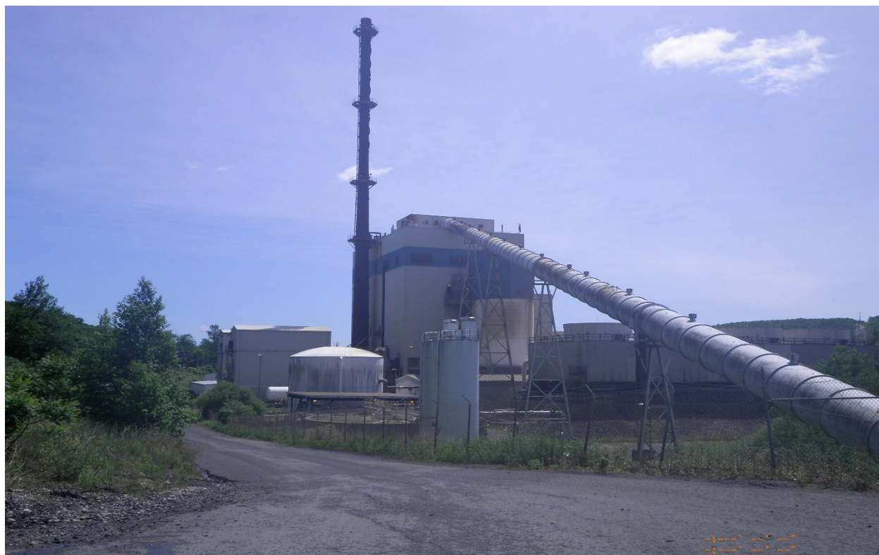
4. Plant and Combined Boiler Stack – Panther Creek Generating – 6/8/22
