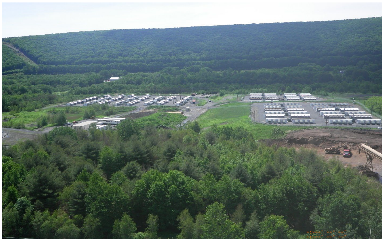
6. Overview of Data Center from Plant – Panther Creek Generating – 6/8/22
