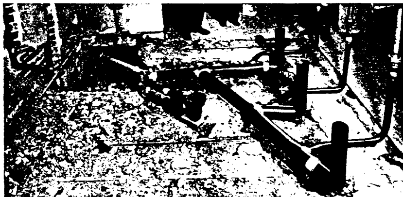
Below, right, lead soil lines in San Antonio, Tex., warehouse toilets.
