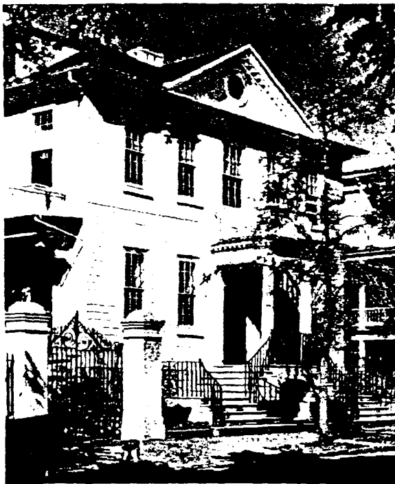
The John Edwards house built about 1800, a fine example of simulated rustication which shows to advantage with the help of pure white lead paint.
