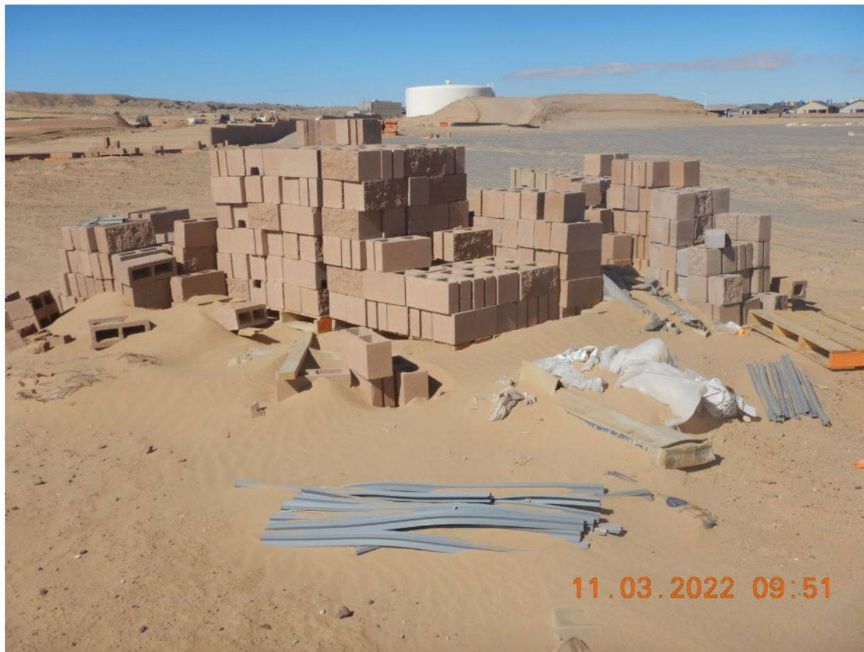
View indicative of unstabilized land surface, i.e., vagrant earthen material. (DSCN2159). Photographed by D. Esparza
