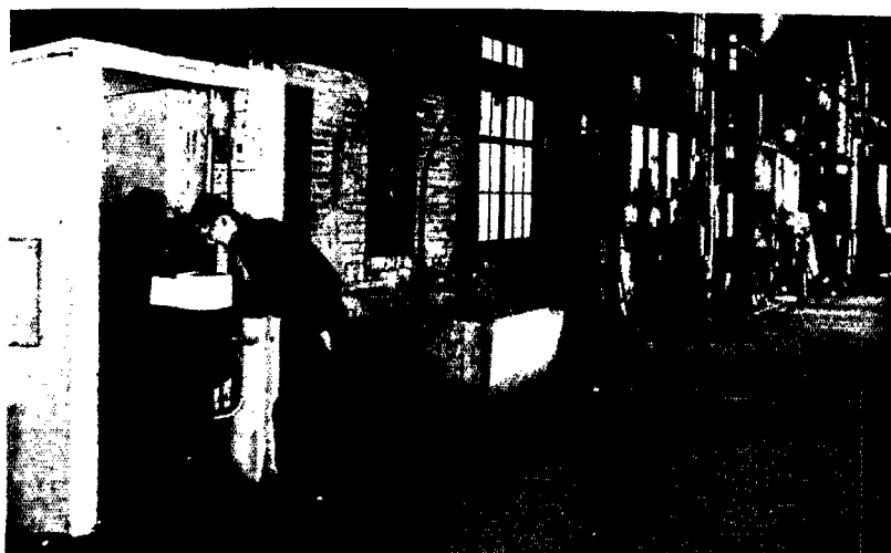
This fountain with a guarded jet which cannot be touched with the lips provides water at regulated temperature. Artificial cooling is usually more economical than leaving a tap running.
