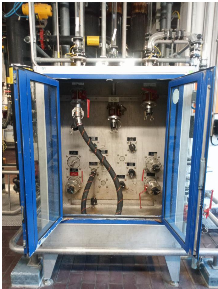
Picture 8 Product distributor with PTFE lined hoses and several sealings
