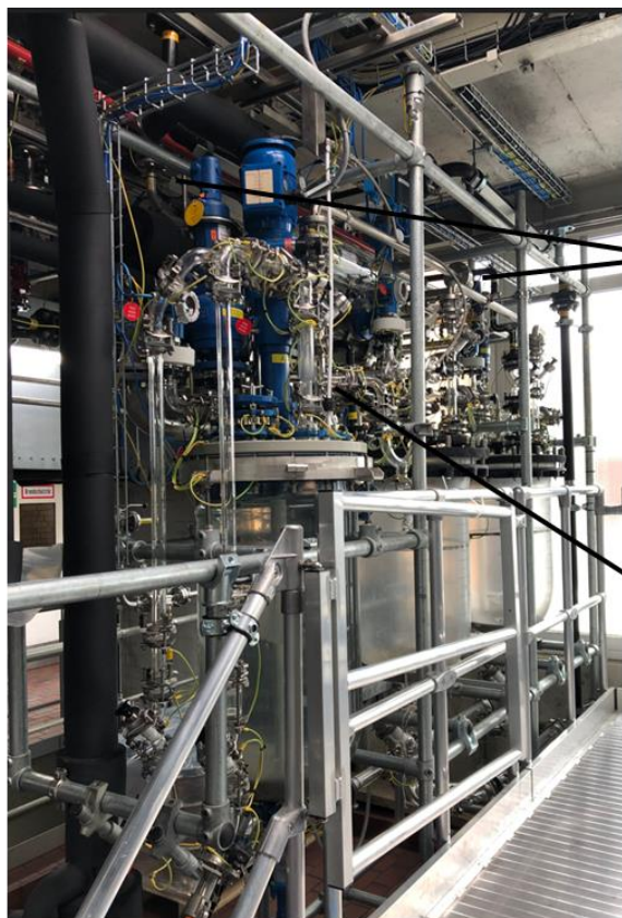
100 L reactor (Glas)
