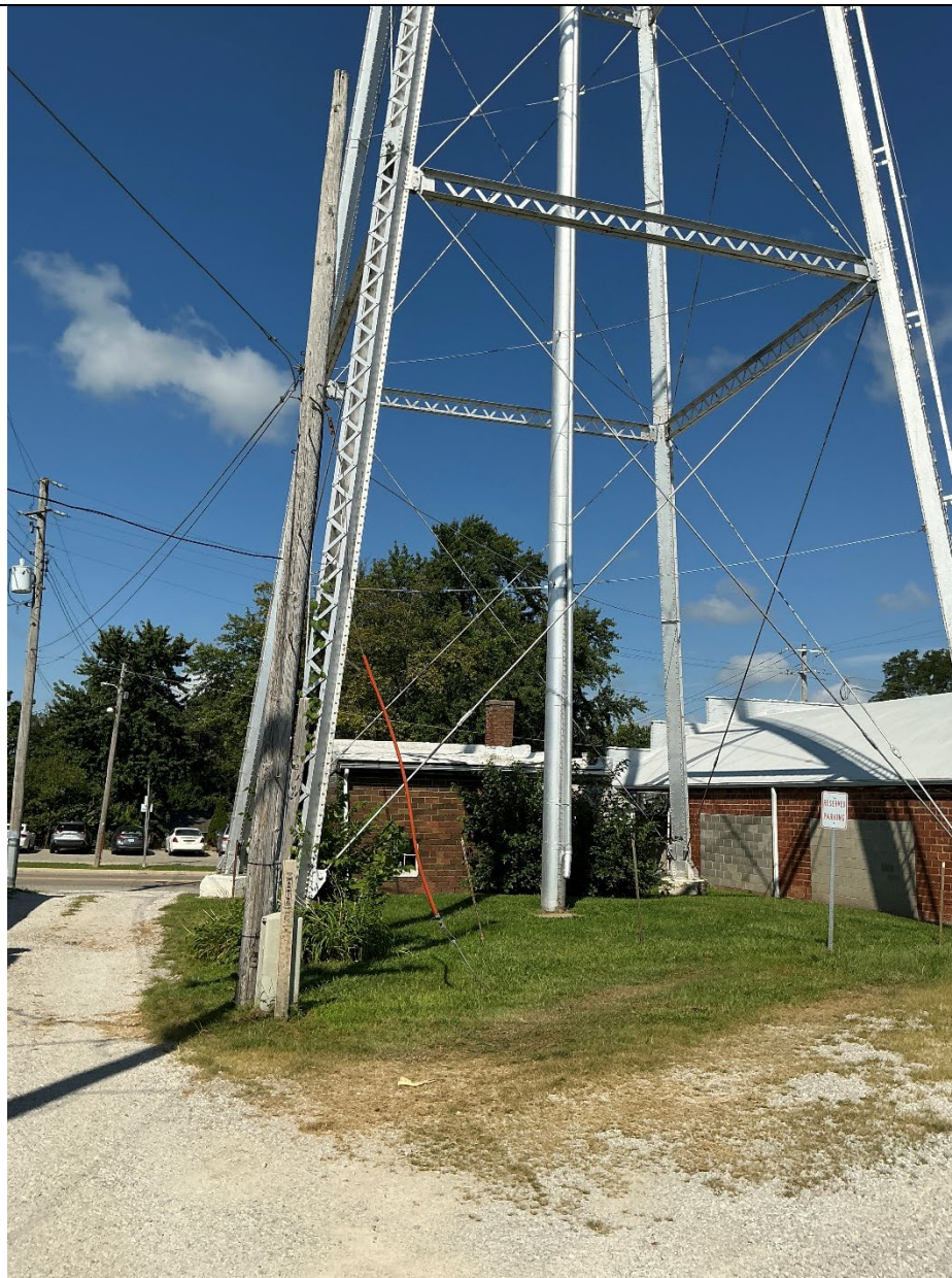
Base of the 75,000-gallon Cone Tower.
