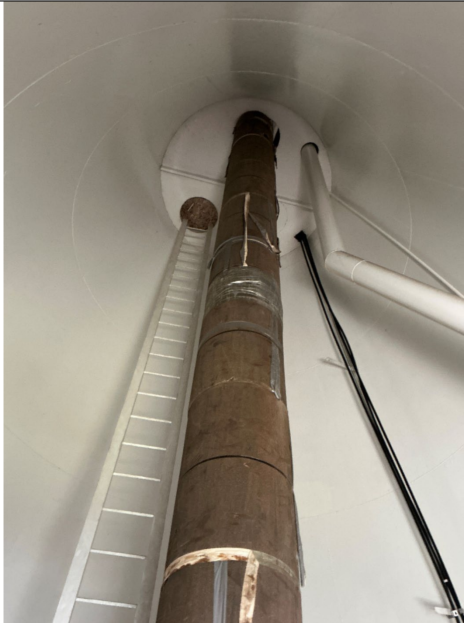
200,000-gallon Sphere Tower interior.
