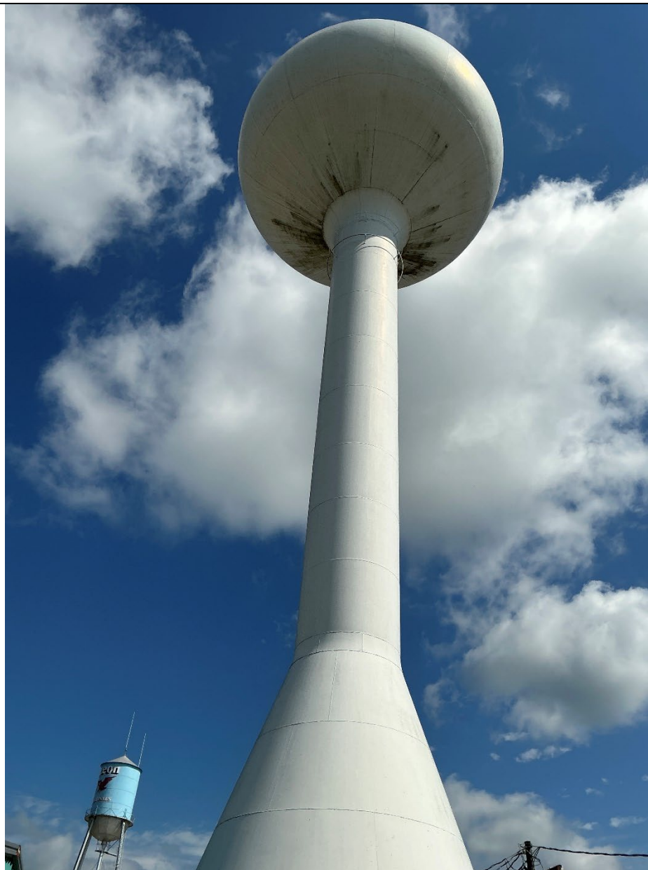
200,000-gallon Sphere Tower exterior.
