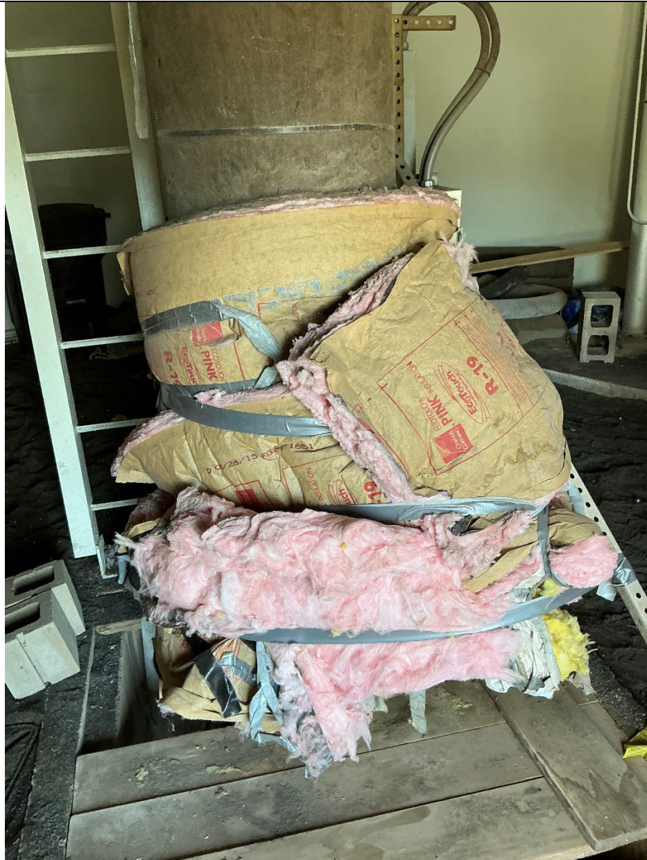
200,000-gallon Sphere Tower interior.
