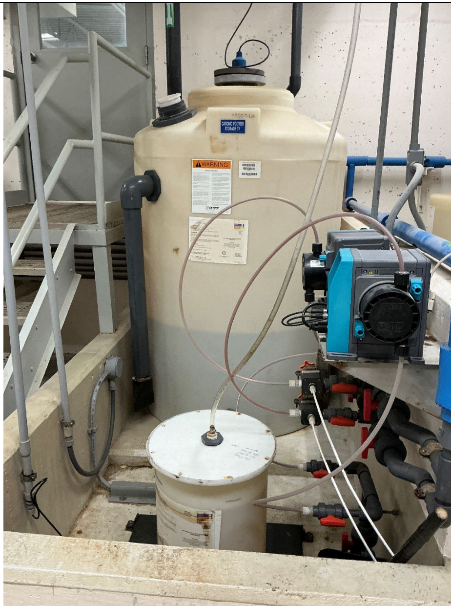
Cationic polymer with secondary containment.
