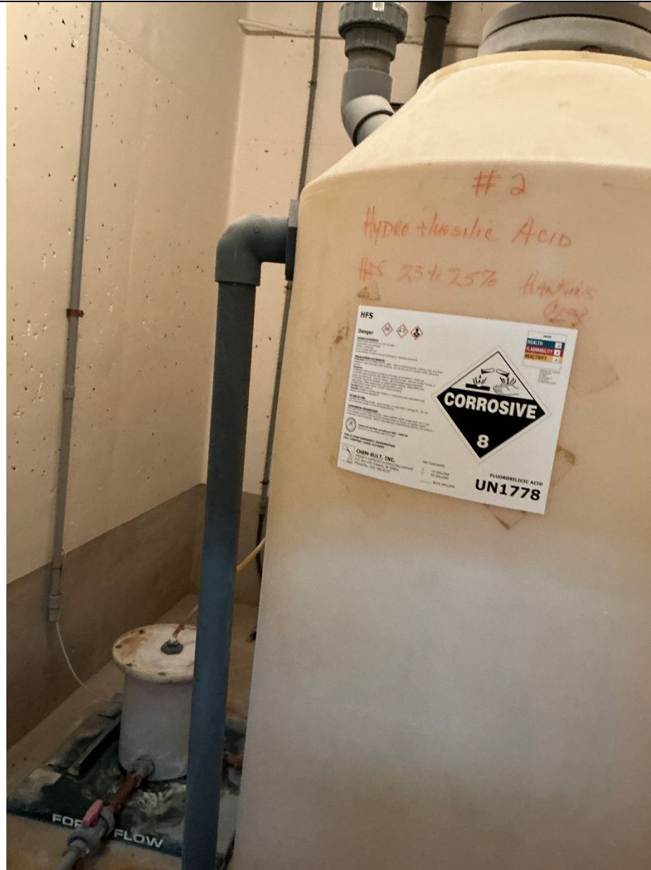
Hydrofluorosilicic acid tank.
