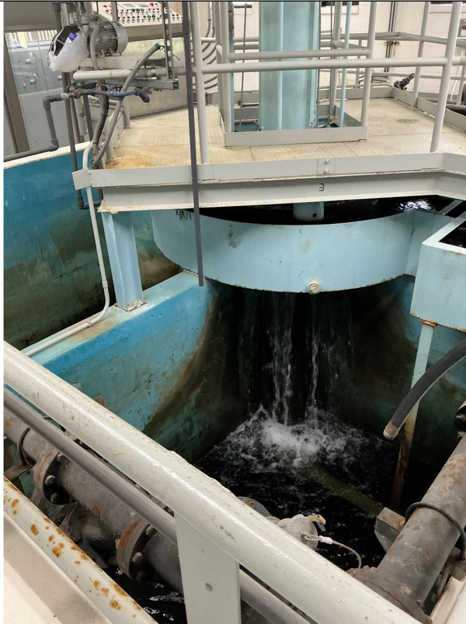
GAC, sand, and gravel filters.
