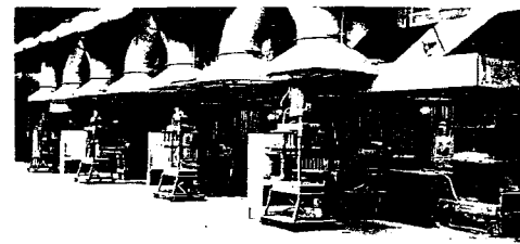
Figure 7. In this foundry, local exhaust hoods are installed over each station having a shell-molding machine and glue press. Adequate make-up air is supplied from ventilating duct situated between molding machines and presses. (Courtesy American Foundrymen's Society)
