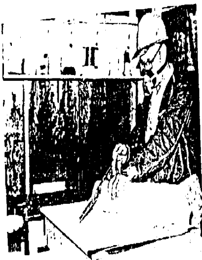
Fig. 3 - Preventing dispersal of asbestos dust by sealing plastic bags containing damp insulation material. The bags are tagged for the delivery site. The materials remain damp for easy installation.
