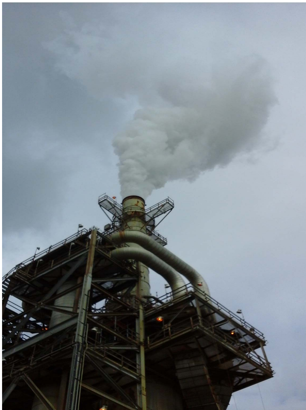
FCCU Wet Gas Scrubber Stack
