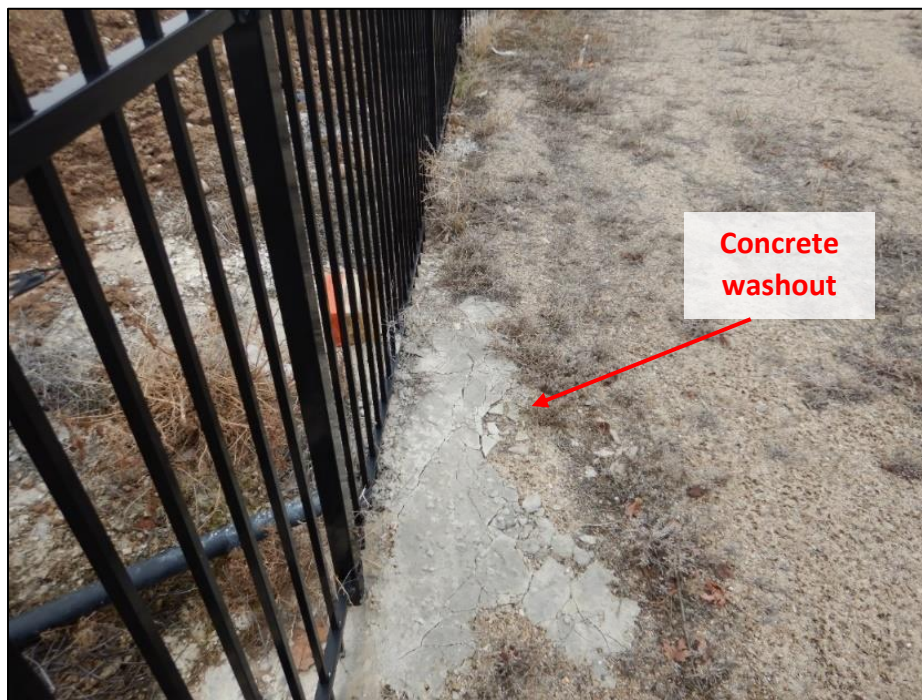
Photograph 9. View, facing south, of concrete washout located along the western perimeter of Phase 5 adjacent to Fivemile Creek. The location is just east of the location shown in Photograph 8 .
