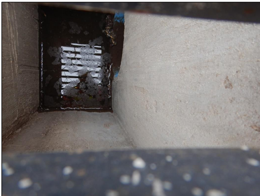
Photograph 7. View inside the storm drain inlet shown in Photographs 5 and 6 . No BMP is located inside the catch basin. The storm drain inlet discharges to a seepage bed in Phase 5.
