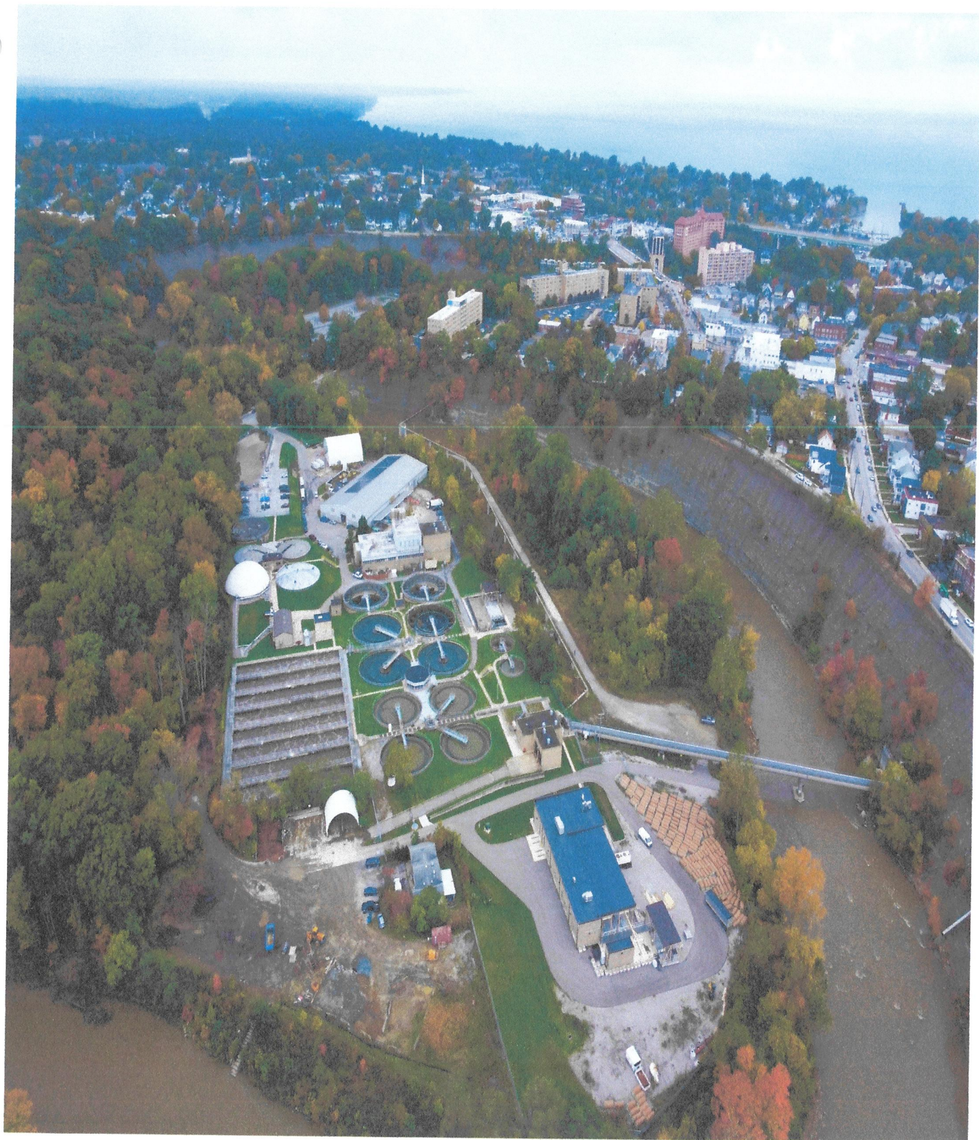
Lakewood WWTP and CEHRT (Chemically Enhanced High Rate Treatment) Plant Aerial View
