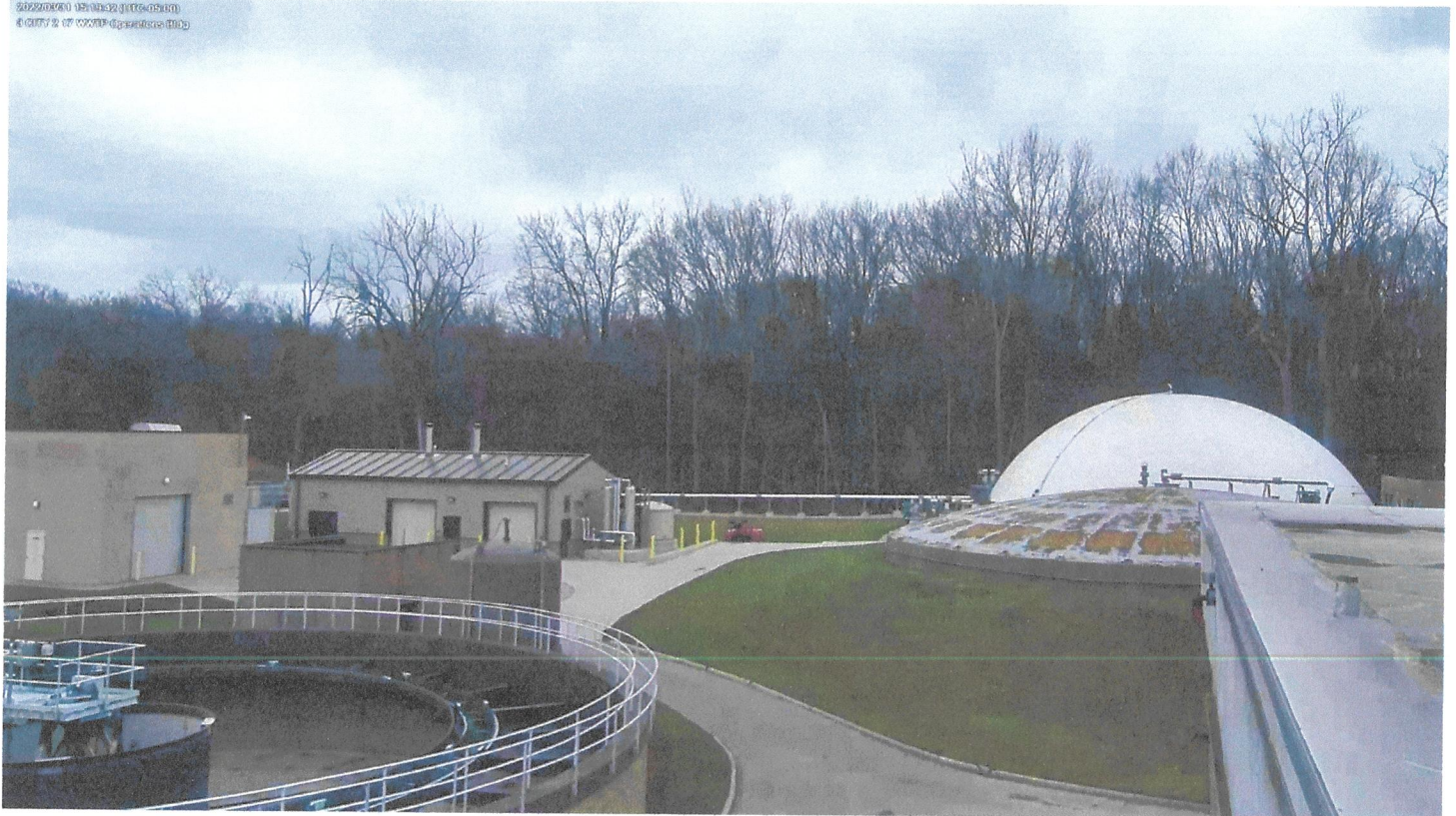
Blowers Building, Energy Recovery Building, and Primary Digesters
