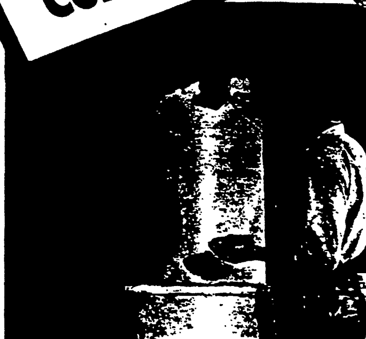
Plisulate Finishing Cement No. 102 is easily applied with a trowel. Photograph above shows the application of No. 102 over Plisulate Insulating Cement No. 101.
