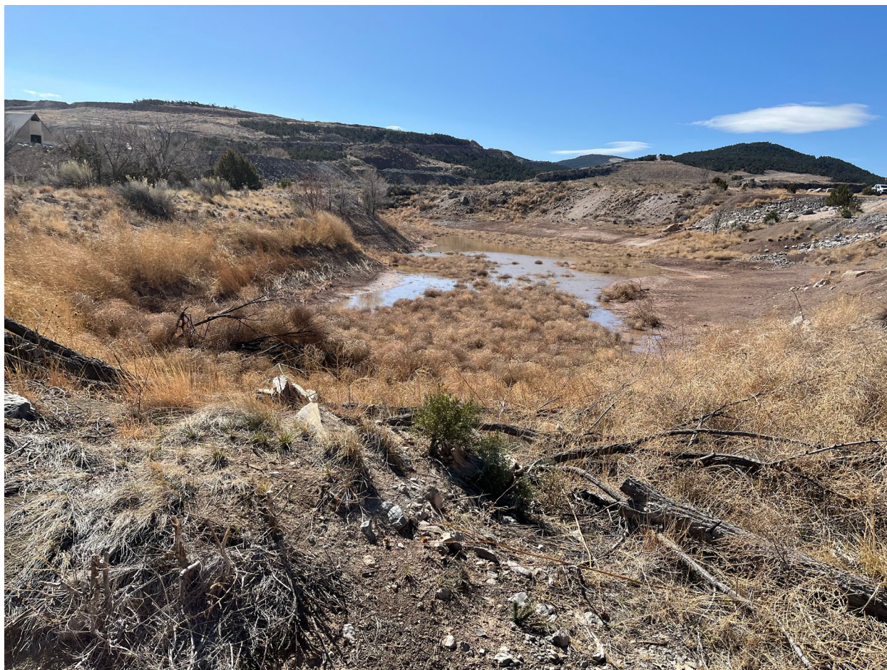
View of the 4M-gallon earthen sediment pond looking approximately Southwest. (IMG_0278). (Photographed 03/12/2025: 10:52 AM) Photographed by D. Esparza
