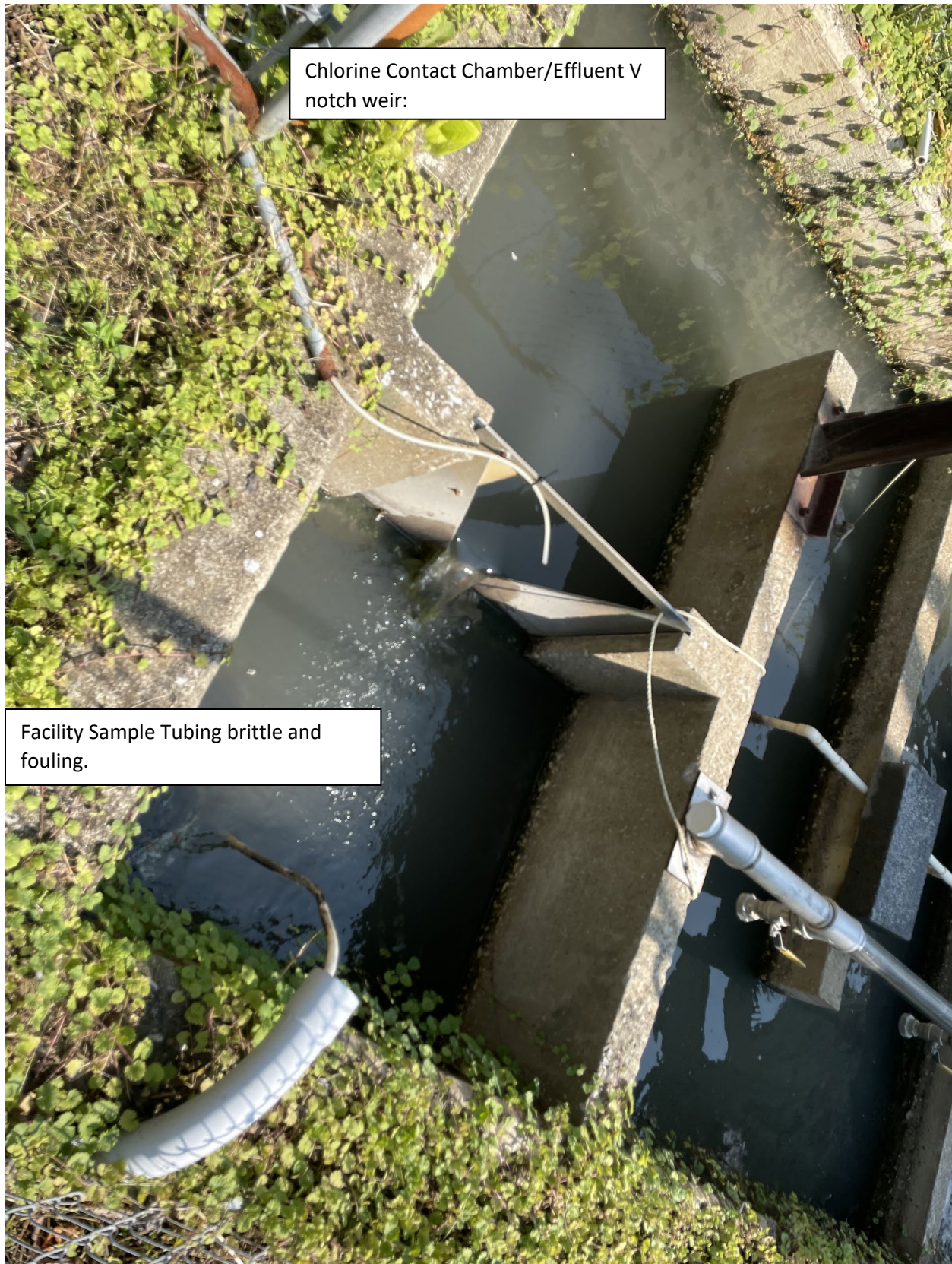
Figure 3: Effluent Discharge Weir photo: Taken 6/13/23 10:12 am
