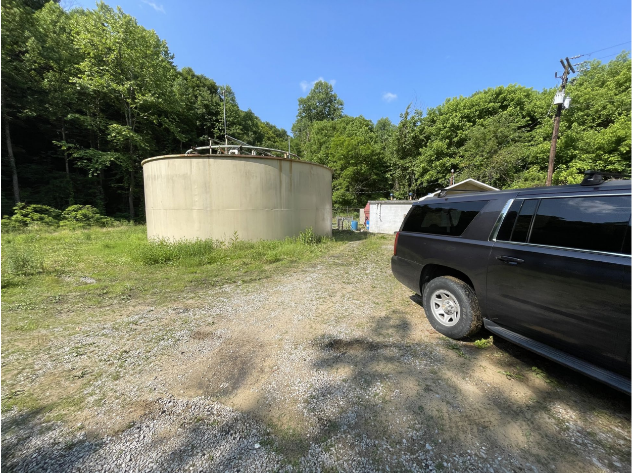
Figure 1: Facility grounds/non-operational clarifier photo: Taken 6/13/23 10:09 am
