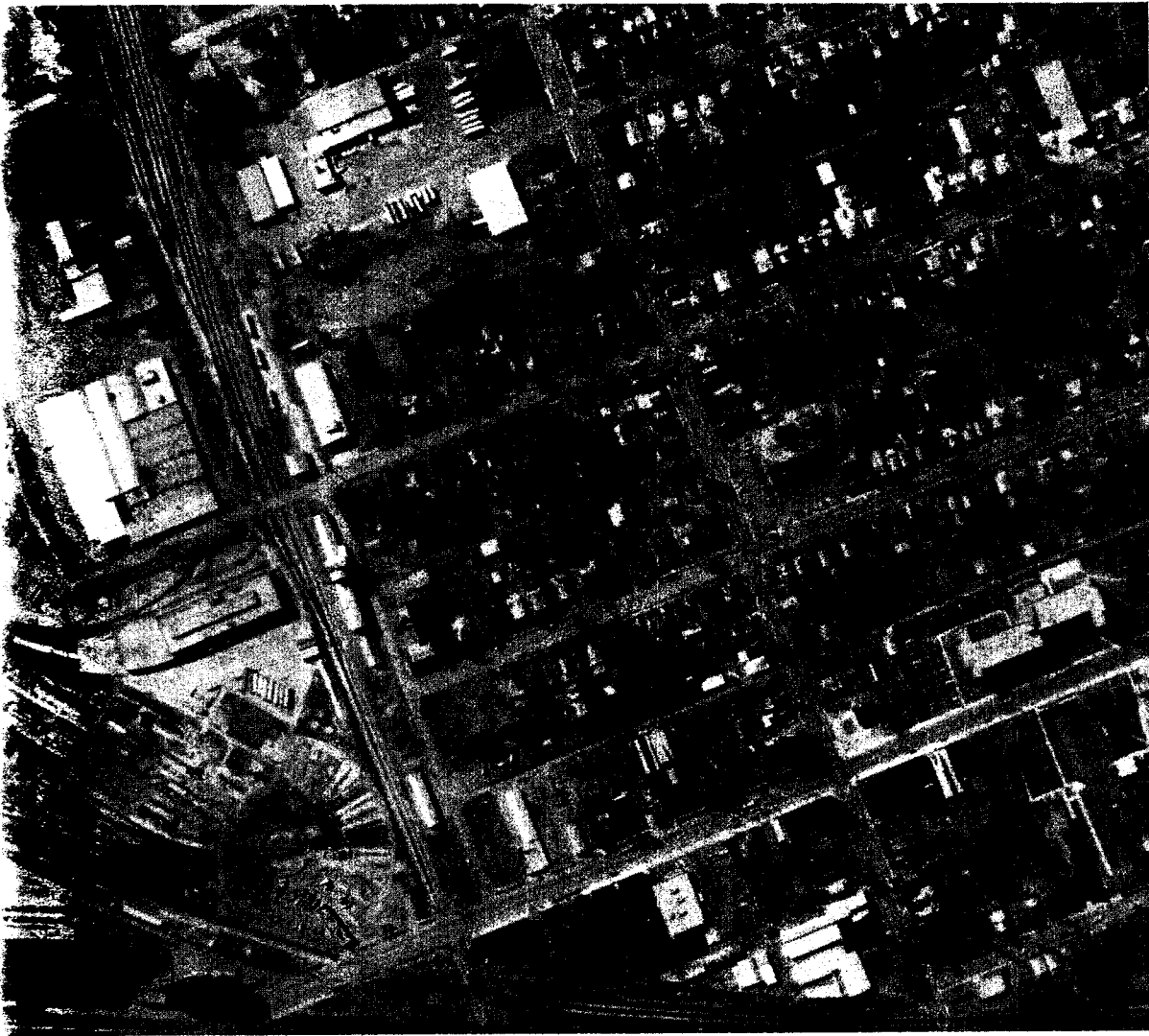
Lima from the air shows clear evidence of the importance of railroading to the community. (City of Lima)
