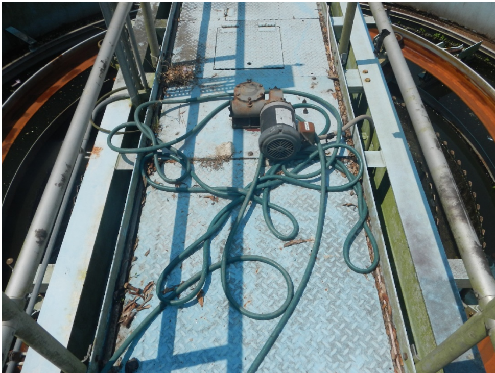
Photo 10: Water hose laid out on aeration tank 2 walkway.
