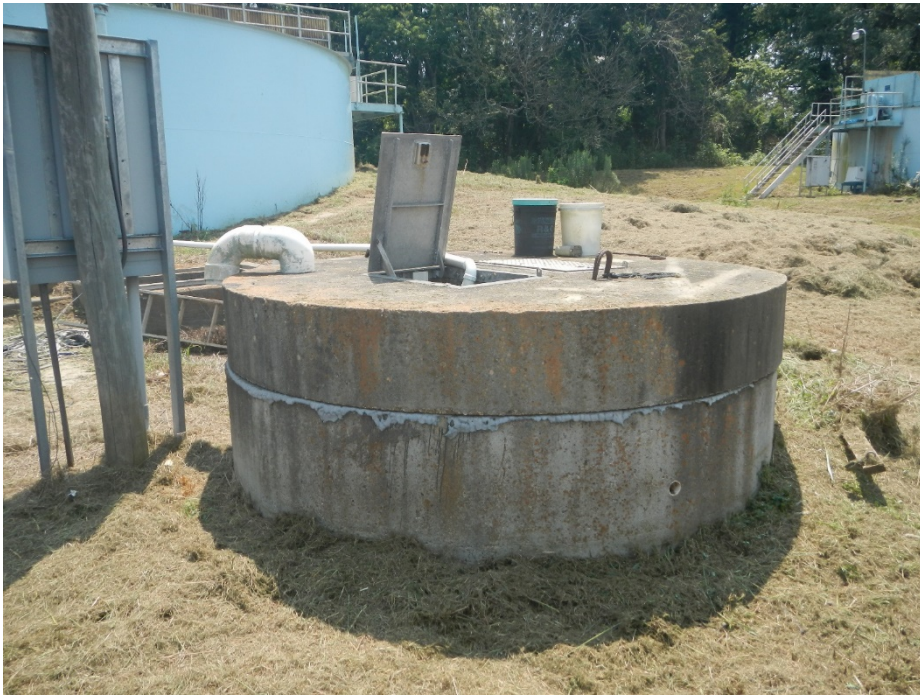
Photo 5: New pump station.
