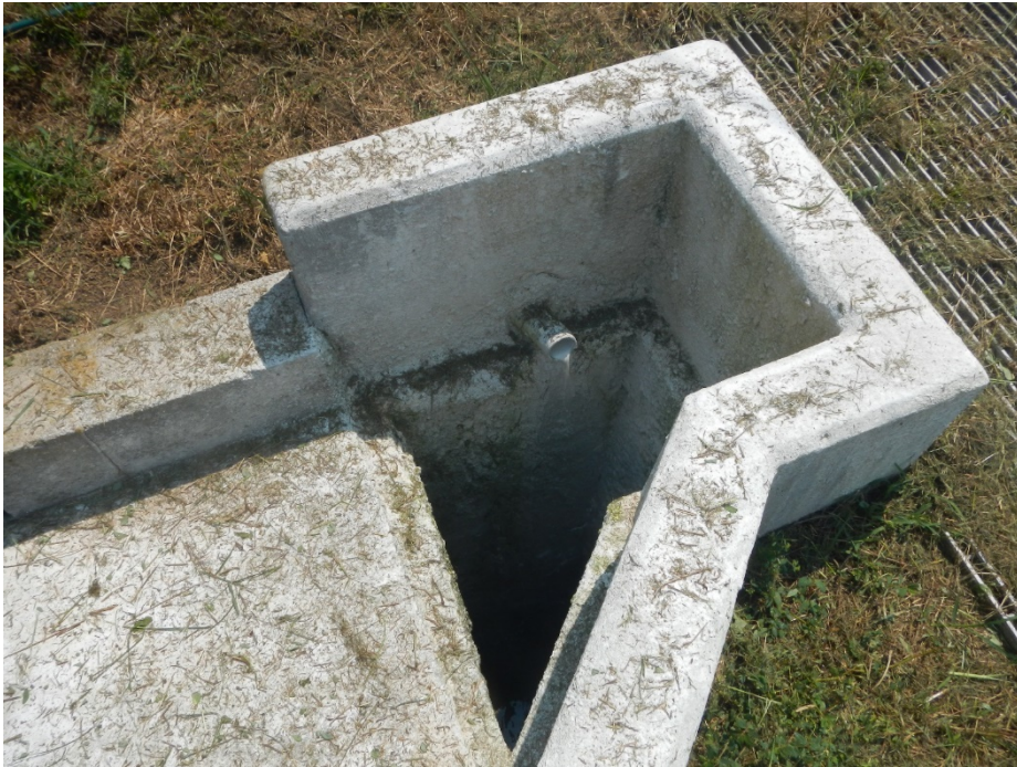
Photo 4: Lime dosing following headworks.
