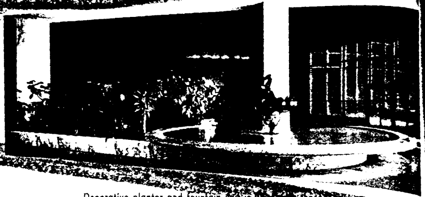
Decorative planter and fountain unit is lined with lead. The lead is exposed in the planter but is an underlayment beneath the fountain tile.
