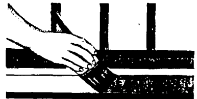
Finish flat surface with long strokes.
