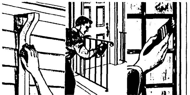
Remove all rust and grease from metal surfaces. Wash where necessary with mineral spirits.
