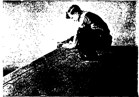
Applying Roll Type Hip and Ridge
