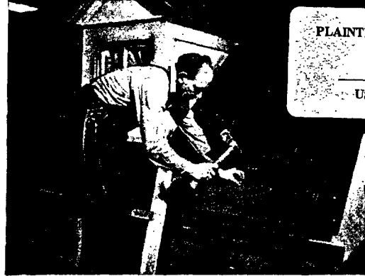
Installing Starter Course
