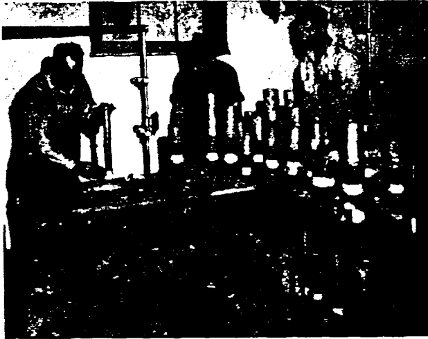
Lead bends and drum traps in a new toilet room in an office building in Tulsa, Oklahoma.
