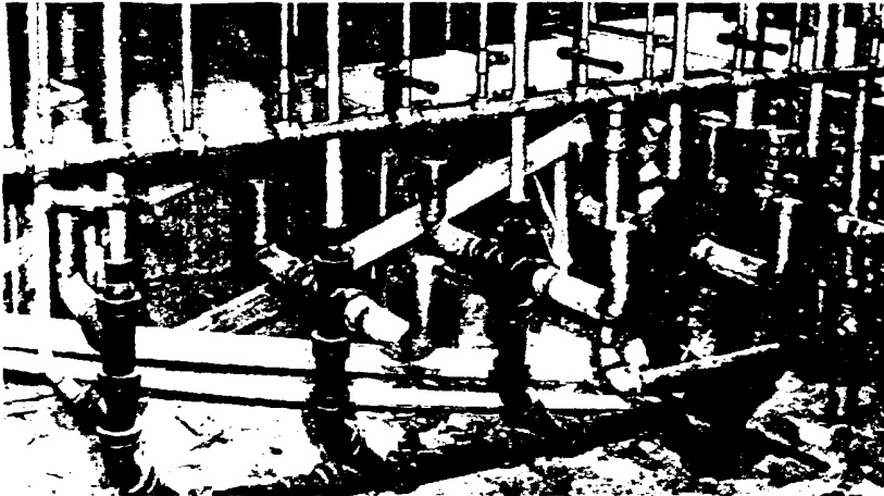
Lead bends and lavatory wastes in toilet room of American Airlines building in Tulsa, Oklahoma.
