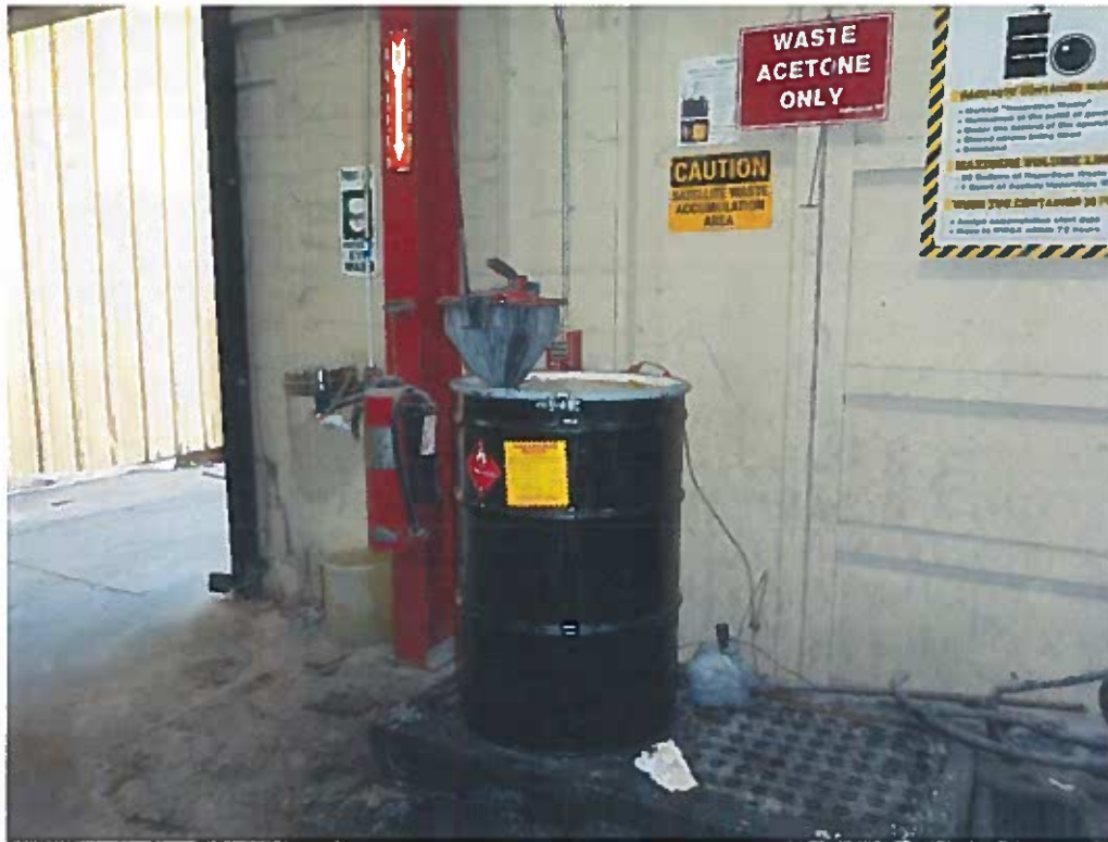
Photo 15: SAA for accumulating waste acetone generated in the winding area within the Light Pole Building.
