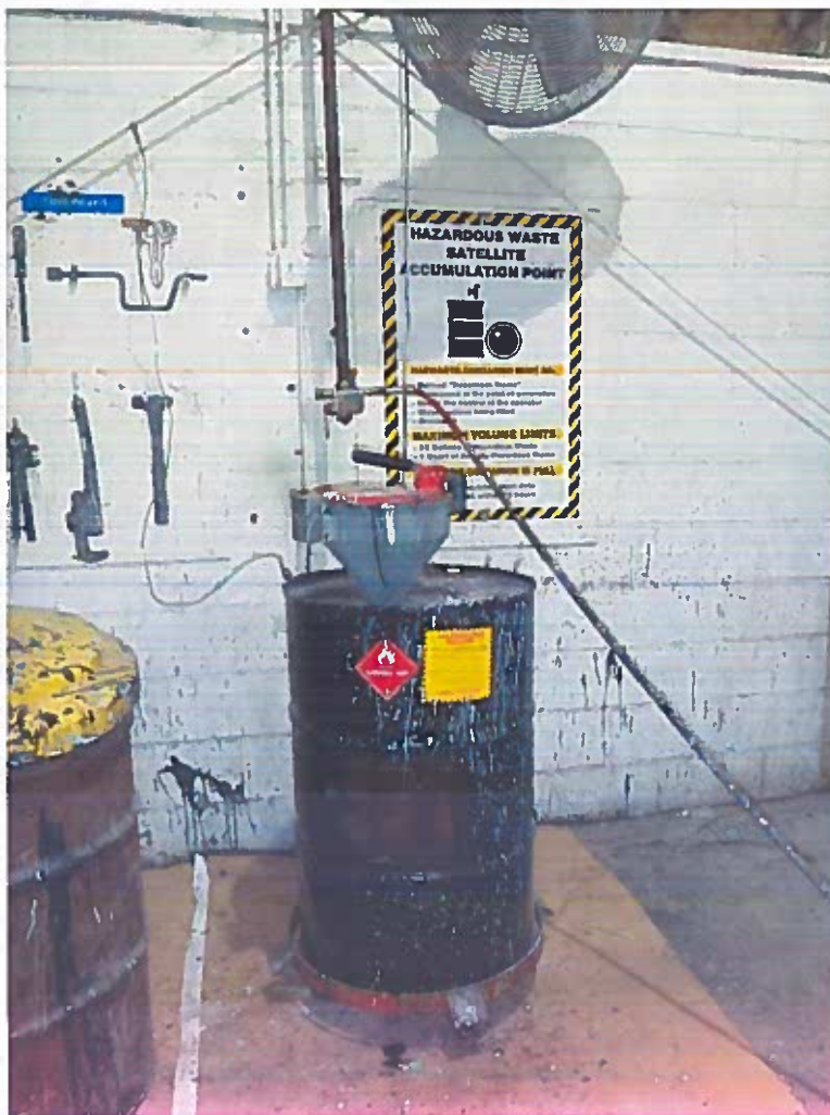
Photo 18: SAA for accumulating waste paint related material generated in the manual painting booths within the Light Pole Building.
