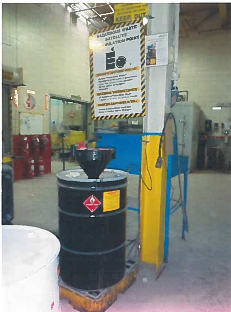
Photo 1: SAA located just outside the Mixing Room for accumulating waste acetone used in cleaning protrusion machines in the Shakespeare area.
