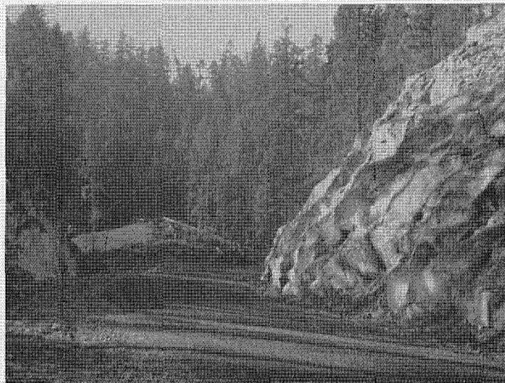
Road Building usually accompanies dam construction. At Hills Creek, dynamite carved West Side Road through stretch of rock.
