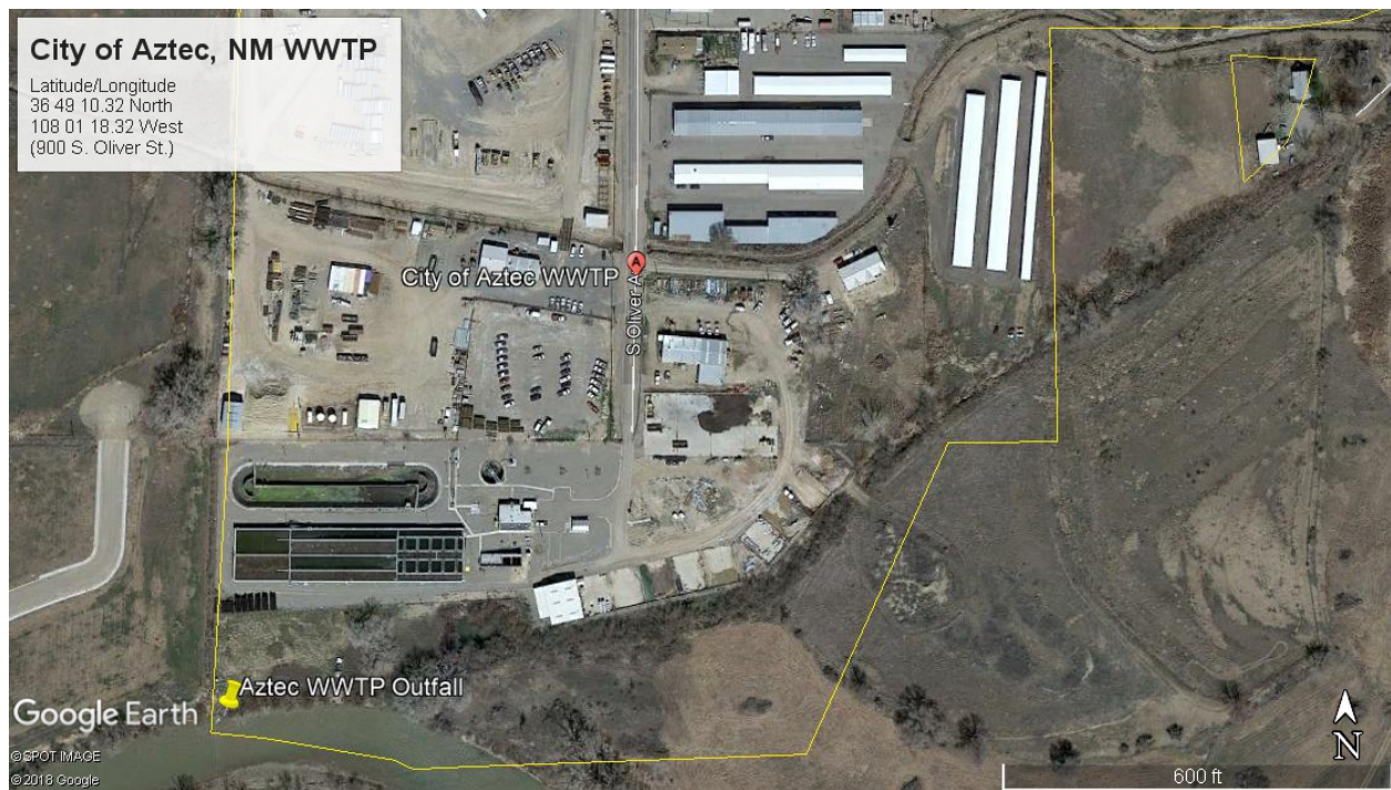
Aerial Image #1: Overall view of the City of Aztec's Wastewater Treatment Plant and Outfall 001. Aerial from Google Earth maps.
