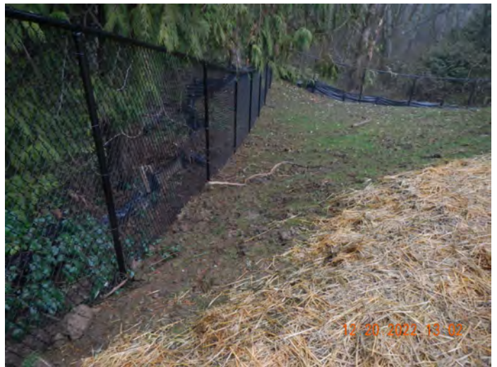
Photo #:28 (DSCN3124) Description: Facing north, photo of area northwest of Pond C.
