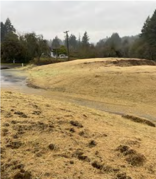
Photo 12a: Along S. 21 st Place, mostly well covered with a few areas lacking enough straw mulch along the fire access road.
