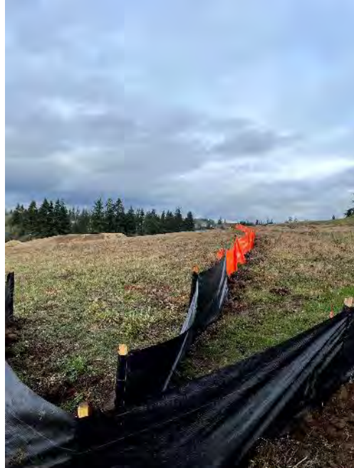
Photo 9b. View of extended and terminated end run of perimeter silt fence along the west side of Phase 5.
