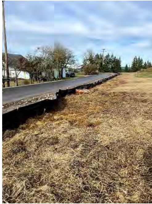
Photo 8b. View facing north of the installed straw mulch and additional silt fence at the entrance to Phase 3, 4, and 5.
