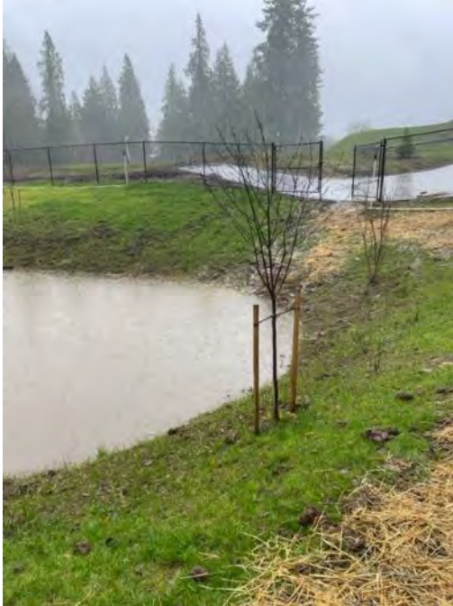
Photo 15a: Pond C entrance area needs maintenance, erosion observed.
