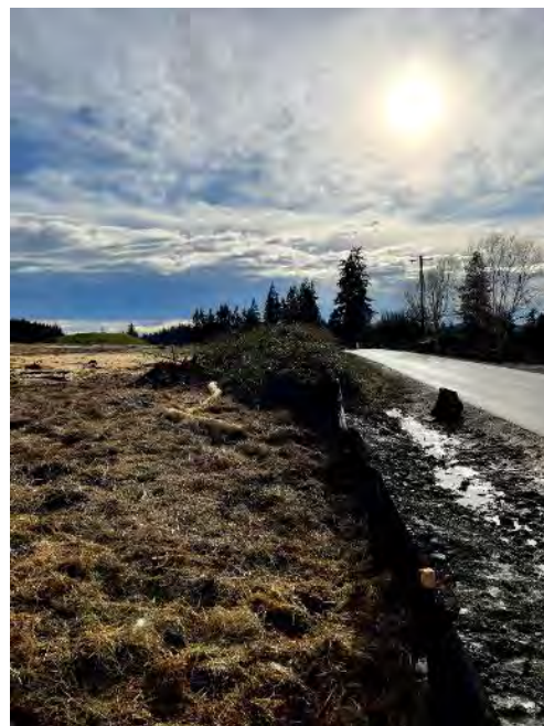
Photo 8d. View facing south of the installed straw mulch and additional silt fence at the entrance to Phase 3, 4, and 5.
