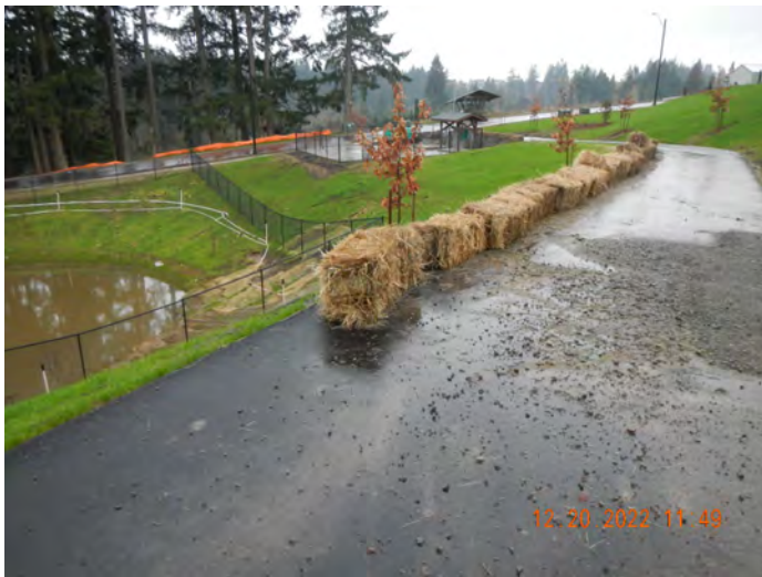
Photo #:11 (DSCN3107) Description: Facing east, photo from above Pond A. Straw bales and conveyance piping installed to assist with run-on to the northern slope of Pond A hillside.
