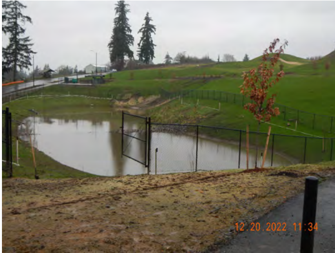
Photo #:05 (DSCN3101) Description: Facing west, photo of Pond A.
