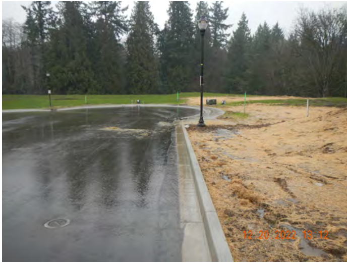
Photo #:31 (DSCN3127) Description: Facing north, photo of the Phase 2 Culdesac.
