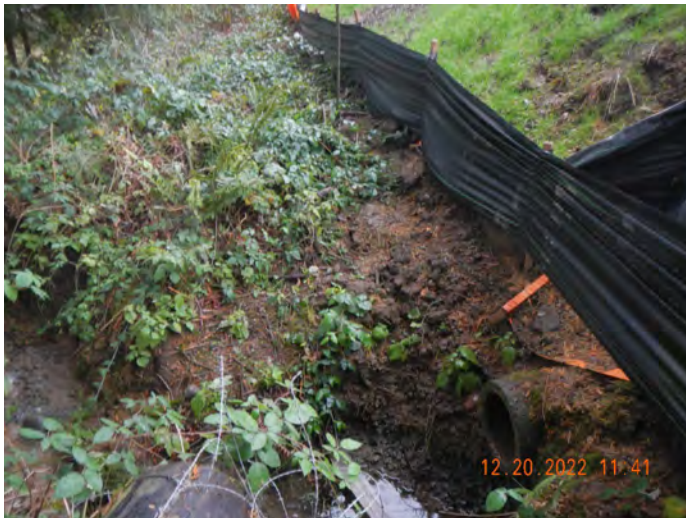
Photo #:07 (DSCN3103) Description: Facing west, photo of outfall pipe from Pond A.
