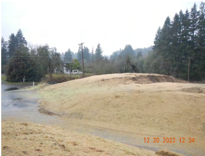
Photo #:23 (DSCN3119) Description: Facing west, photo of fire access road and stockpiles within Phase 5.
