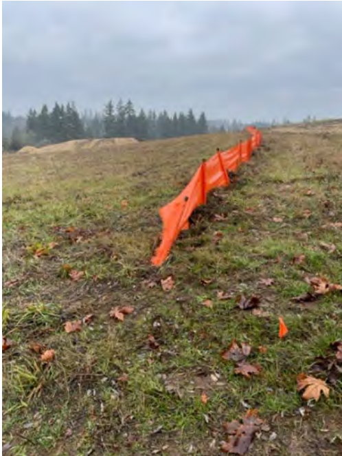
Photo 9a. West side of Phase 5 Silt fence needs to be extended.
