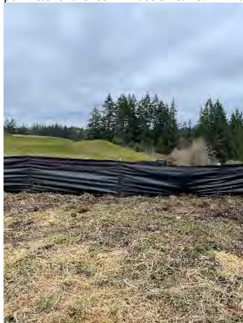
Photo 10b – View of installed straw mulch stabilization and perimeter silt fence in Phase 5 near S. 4 th Way.
