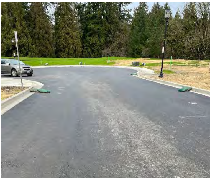
Photo 17c – View of curbside check dams installed in the Phase 2 cul-de-sac.
