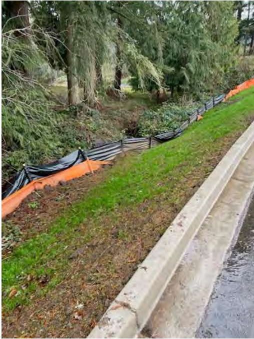
Photo 3a: Silt fence at Pond A discharge needs maintenance.
