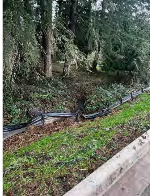
Photo 3b: View of maintained perimeter silt fence adjacent to the Pond A discharge pipe.
