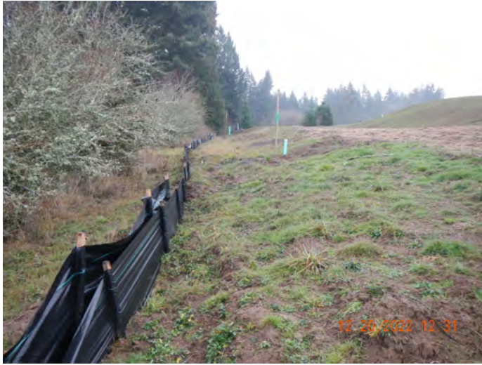
Photo #:21 (DSCN3117) Description: Facing east, photo of northern perimeter silt fencing
