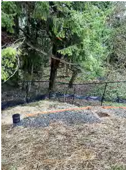
Photo 13b: View of maintained silt fence along the north perimeter of Pond B.
