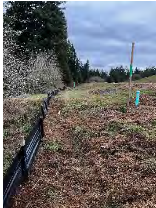
Photo 11b: View of maintained perimeter silt fence along the northwest corner of Phase 5.
