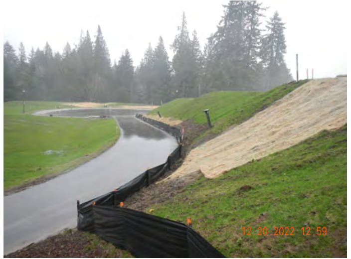
Photo #:26 (DSC3122) Description: Facing east, photo of area east of Pond B and west of Pond C.
