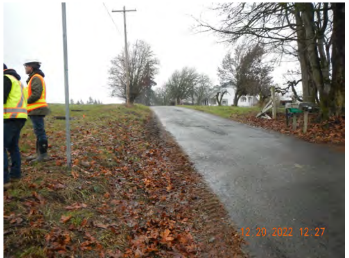
Photo #:20 (DSC3116) Description: Facing east photo of the uncleared areas/perimeter north of S. 25 th Place.
