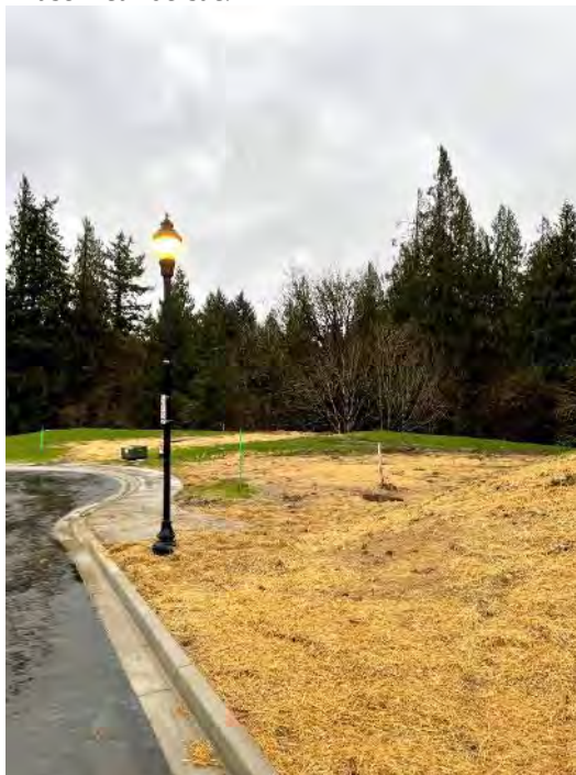
Photo 17b: View of additional straw mulch installed along the Phase 2 cul-de-sac.
