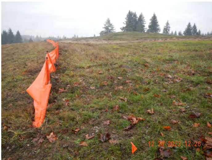
Photo #:19 (DSCN3115) Description: Facing north, perimeter silt fencing along the northwest perimeter.
