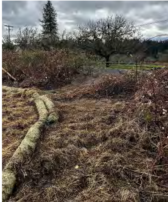
Photograph 7b. View of installed straw wattle and straw mulch at the low point along Phase 3 perimeter at S. 25 th Place.
