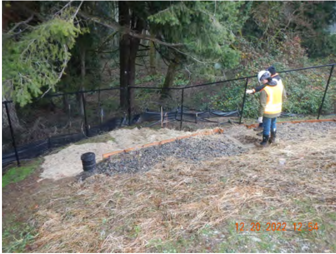
Photo #:25 (DSCN3121) Description: Facing north, photo of Pond B. outfall location.
