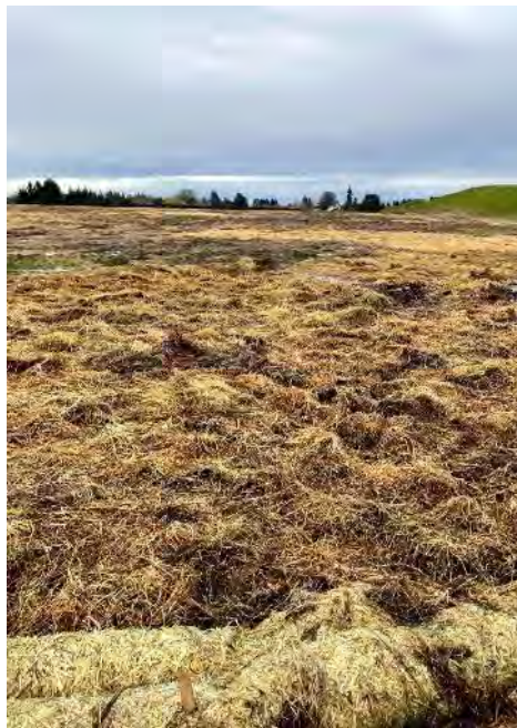
Photo 18b: View of installed straw mulch stabilization in Phase 3.
