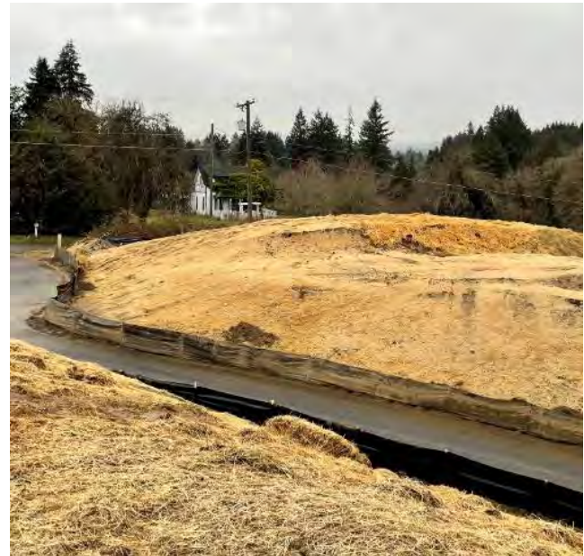
Photo 12b: View of additional mulch and perimeter silt fence installed along S. 21 st Place and the fire access road.
