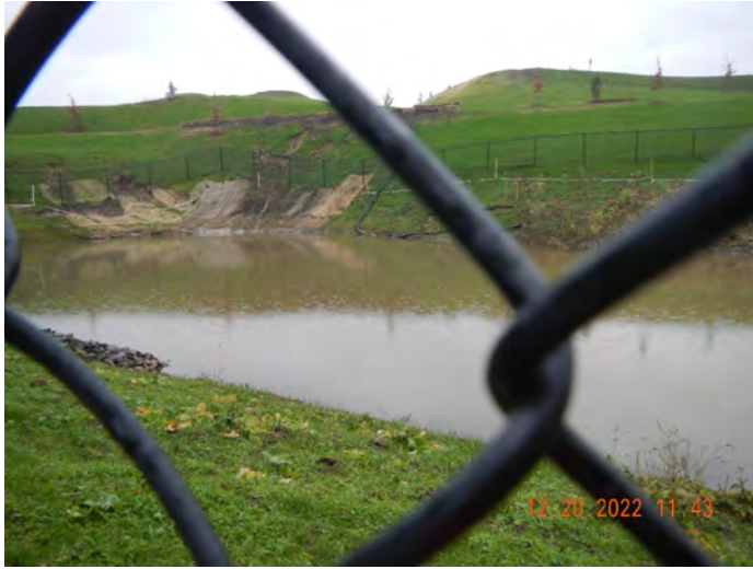
Photo #:09 (DSCN3105) Description: Facing north of Pond A.
