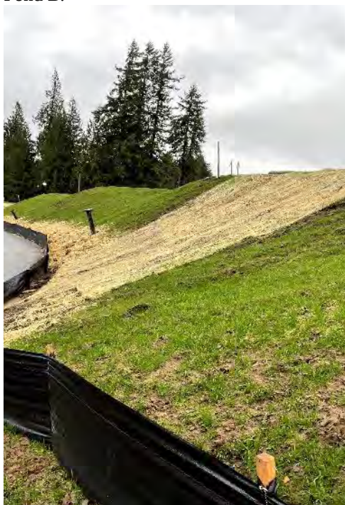
Photo 14b: View of maintained silt fence and additional straw mulch installed on the north side of the footpath and Pond B.
