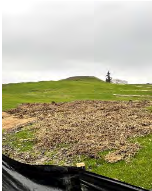
Photo 6d: View of straw stabilization and linear straw wattles installed.
