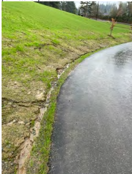
Photo 5a: Path by Pond A has some erosion along the perimeter of paved area.
