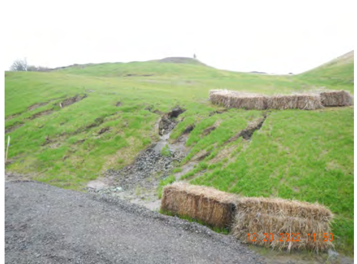
Photo #:12 (DSCN3108) Description: Facing west, photo from above Pond A. Straw bales and conveyance piping installed to assist with run-on to the northern slope of Pond A hillside.
