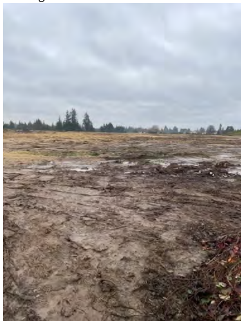
Photo 18a: Phase 3 exposed soil needs straw coverage.
