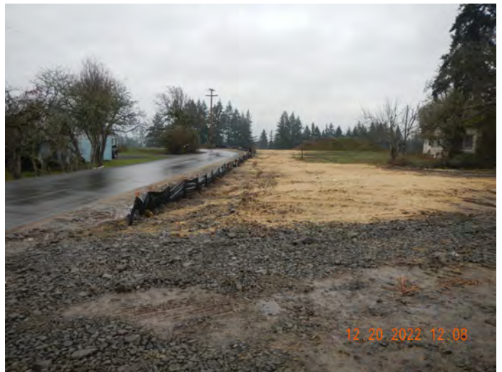
Photo #:16 (DSCN3112) Description: Facing north, photo of an entrance to Phase 3 along S. 25 th Place.
