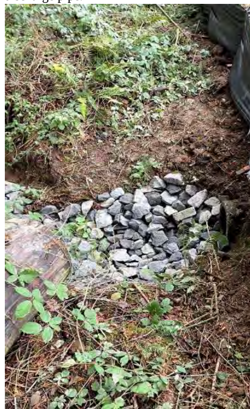
Photo 4b: View of installed outlet protection at Pond A discharge pipe.
