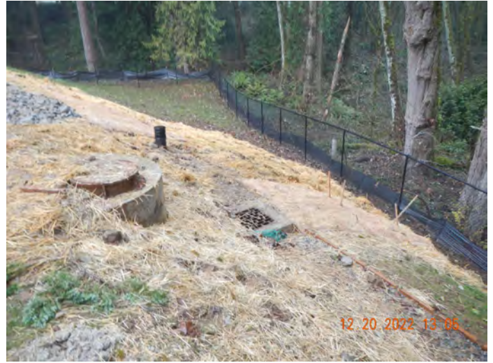
Photo #30: (DSC3126) Description: Facing west, photo of the Pond C outfall area.
