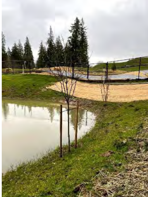
Photo 15b. View of installed erosion control matting on the south slope of Pond C.
