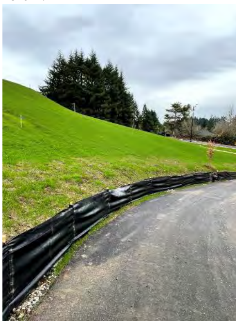
Photo 5b: View of installed silt fence along the footpath at Pond A.
