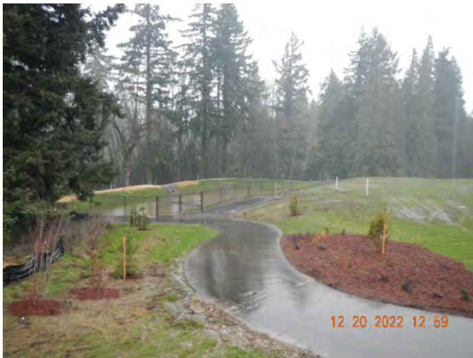
Photo #:27 (DSCN3123) Description: Facing northeast, photo of access road to Pond C.
