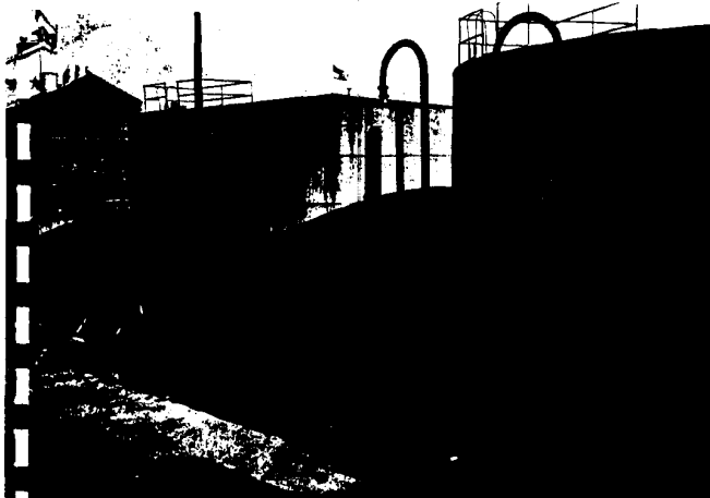
Molasses storage tanks of the New England Alcohol Company.
