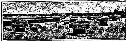
Effico Rotary Ball Bearing Ventilator Installation, Wind Driven (only) The Effico Wind Electric Also as the Same Artistic Lines and Pleasing Appearance. Lowest in Height of Rotary Ventilators by Over 50 per cent Average.
