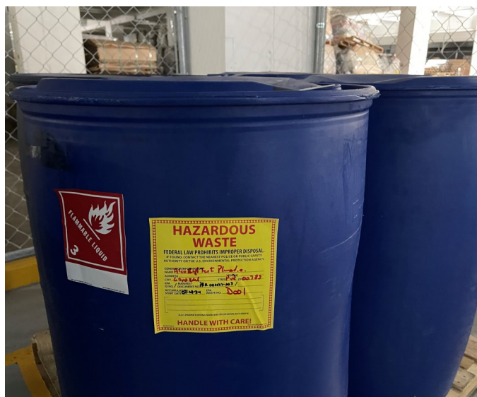
Picture 12 - ALCO HIGH TECH PLASTICS - At the 90-day Hazardous Waste Accumulation area, I observed seven (7) 55-gallon blue plastic drums containing with spent liquid solvent waste containing a mixture of propanol mix 80/20 and ink waste and coded as “D001” (Ignitable). All drums were clearly labeled with the words, “Hazardous Waste,” and dated Feb-Mar 2024.
