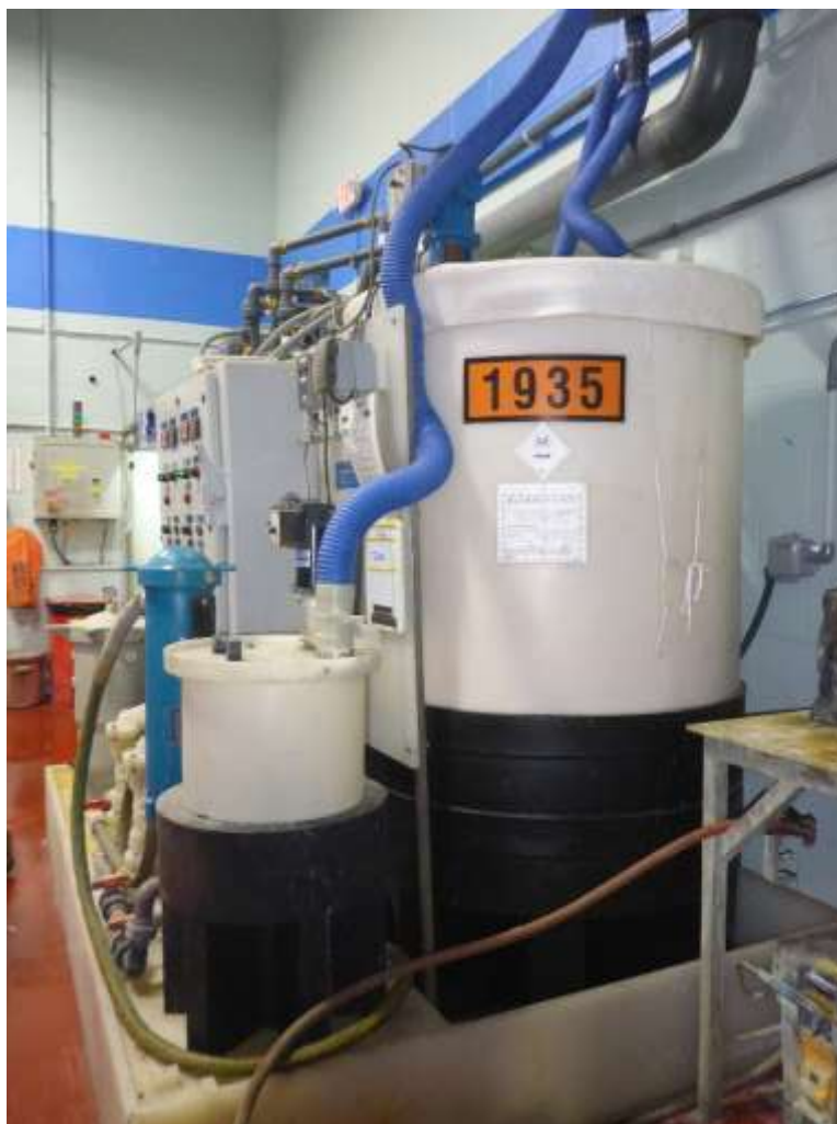
Photo 11: One of two 500-gallon storage tanks for managing hazardous waste liquids that contain precious metals inside the chemical storage area.
