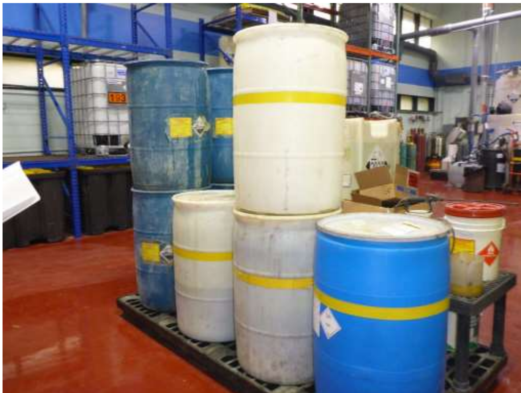
Photo 12: Two portable secondary containment pallets holding ten 55-gallon drums on the floor toward the center of the chemical storage area room.
