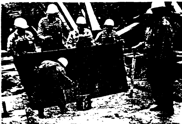
Workmen apply asphaltum to pad before installation . . . and position pad to receive base plate.
