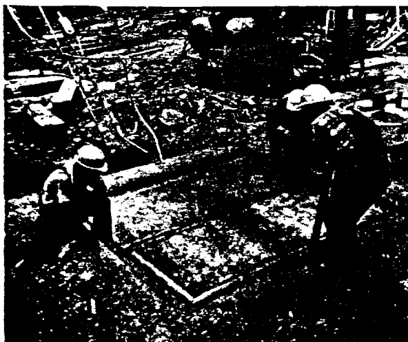
Workmen apply asphaltum to pad before installation . . . and position pad to receive base plate.
