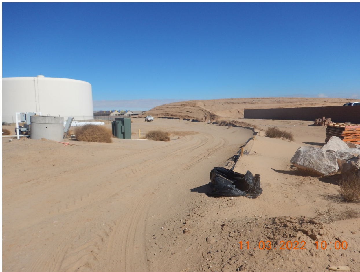
View of stockpiled unstabilized "cut" (earthen material) located along the east side of the Village of Los Lunas WST. Note: the height of the staged material in comparison to the vehicle and WST. (DSCN2163). Photographed by D. Esparza
