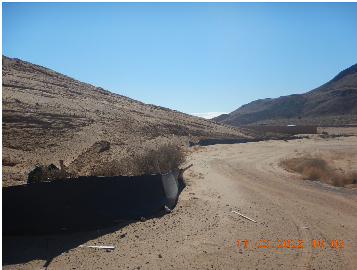
View of stockpiled unstabilized "cut" (earthen material) located along the east side of the Village of Los Lunas WST. (DSCN2165). Photographed by D. Esparza
