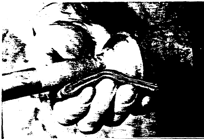
Wiping a solder joint between a lead alloy cable sleeve and a lead alloy sheath.
