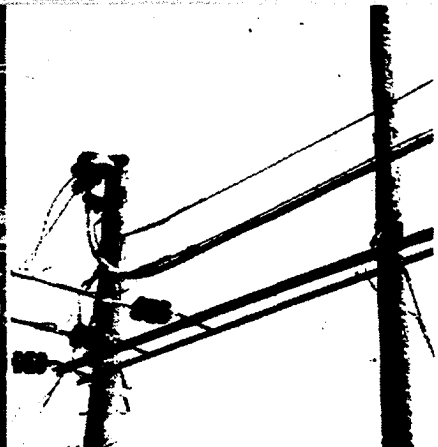
Top. A cable train burying lead sheathed coaxial cable for cross-country communication. Left. Inside a manhole, showing the variety of lead sheathed power cable carried in conduits beneath city streets. Right. Overhead 23,000-volt lead sheathed power cable and terminating pot head.
