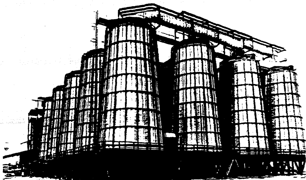
Mills-Packard chambers for making sulphuric acid. They are constructed entirely of sheet lead supported in a steel frame and cooled externally by water flowing down the sloping sides.
