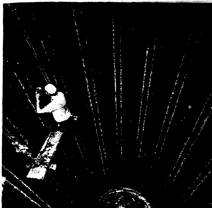
Welding a vertical lap seam on the lead strap covers of a steel strapped lead lined foamite tank.
