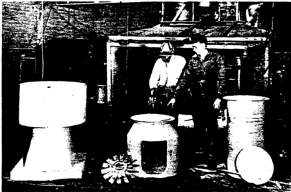
Spraying pure lead on parts of a sheet metal exhaust system to be used for venting sulphuric acid fumes.
