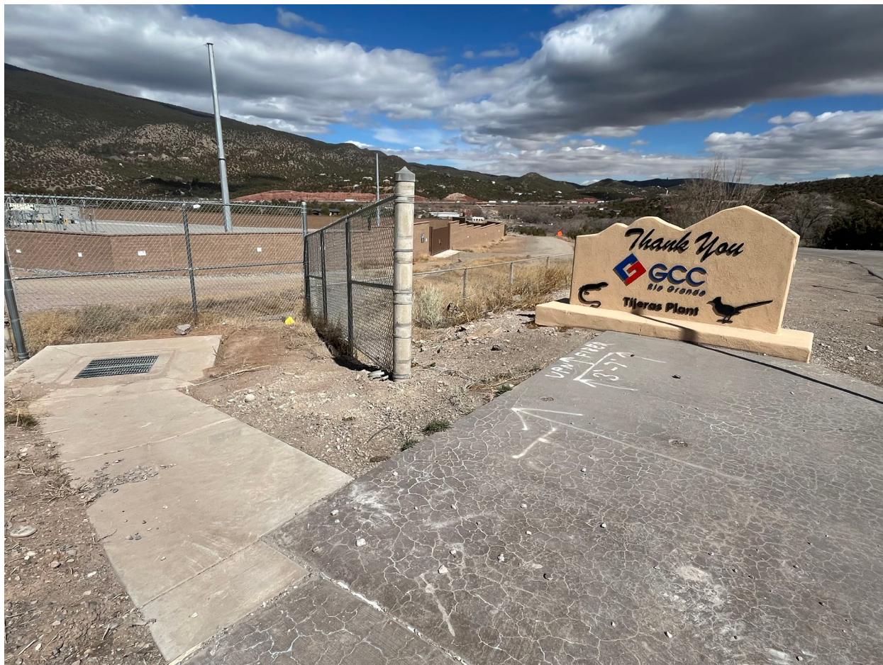
Another view of the drop drain at Outfall 002 looking approximately Northeast. Note: the slope towards the drain. (IMG_0281). (Photographed 03/12/2025: 12:01 PM) Photographed by D. Esparza
