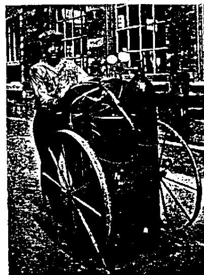
Figure 3. A cart for transporting welding equipment.
