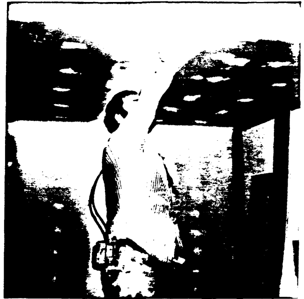
4 (b) Sanding ceiling tape-joints
