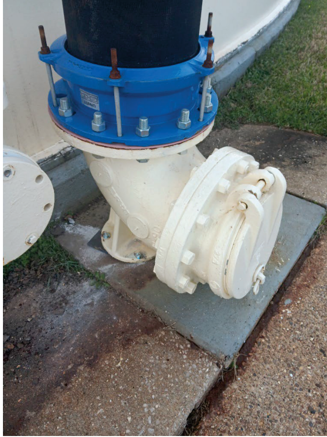
Overflow pipe at 1.0-MG storage tank at Plant 4 secured to the concrete pad. This photograph addresses Observation 11.
