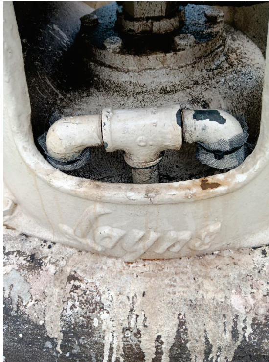
Vent screens replaced on Well #2. This photograph addresses Observation 4.
