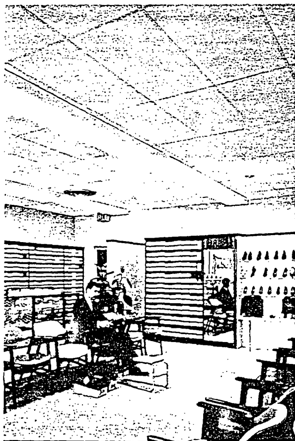
PERFECT BALANCE between sound absorption and attenuation keynotes AURATONE mineral fiber ceiling panels. Grid system offers access to plenum areas. This is the Star pattern, one of six available. Bono's Shoe Store, St. Louis, Mo.; Architect: Charles O'Keefe.
