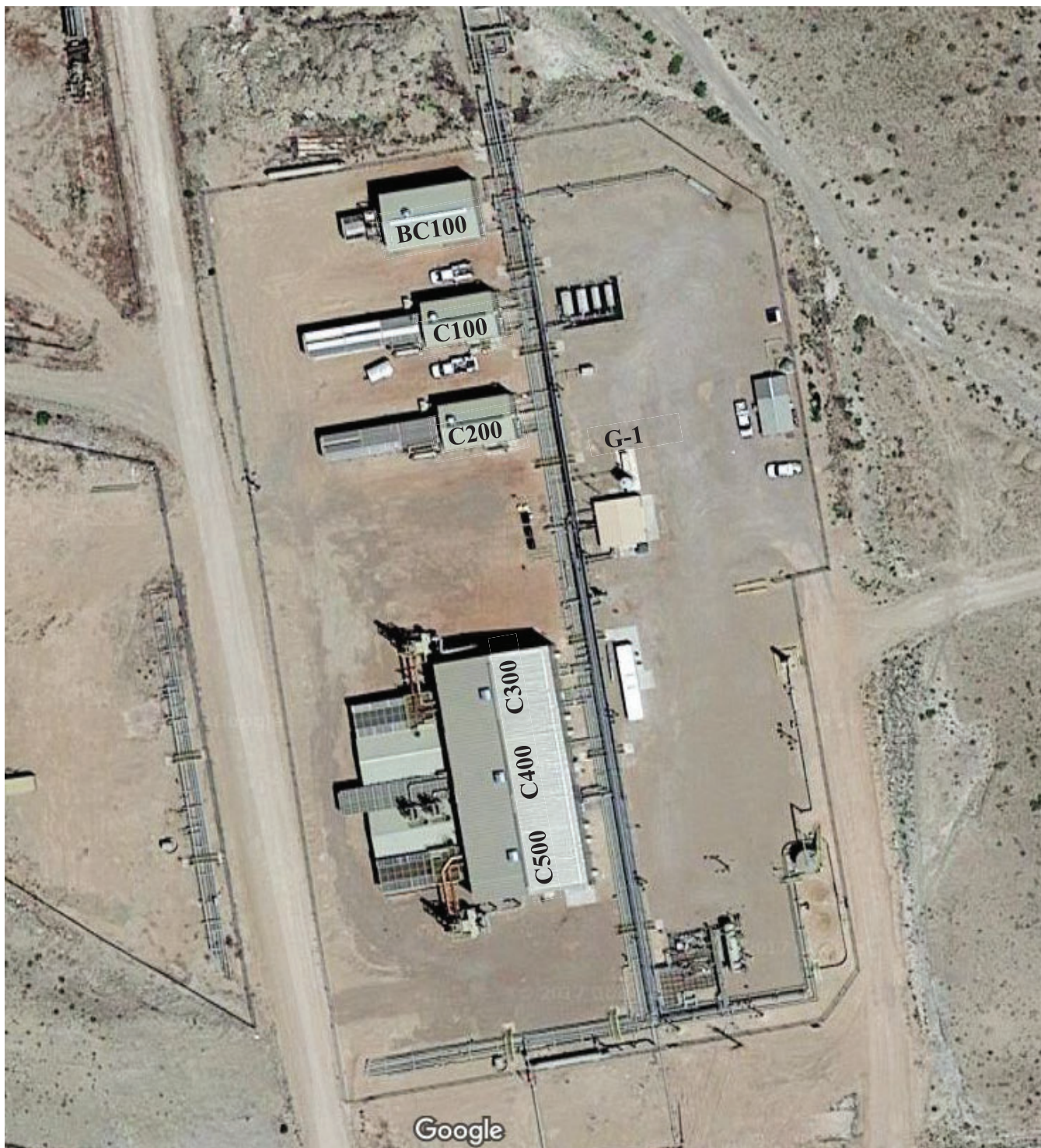
Figure 1: Coyote Wash Compressor Station Aerial View
