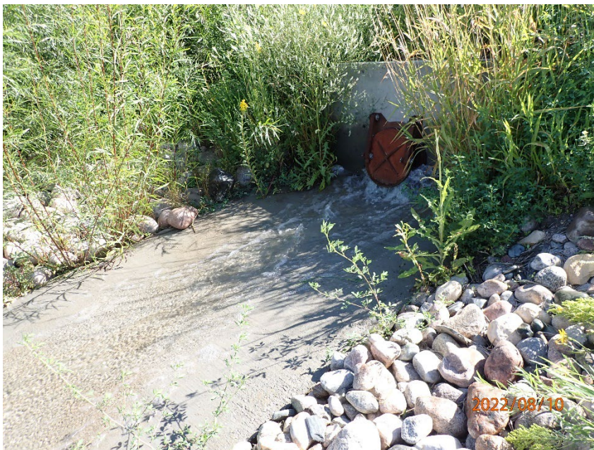
7: P8100031 Description: Discharge Sample Location Location: Waubun WWTF Camera Direction: NE Date/Time: August 10, 2022
