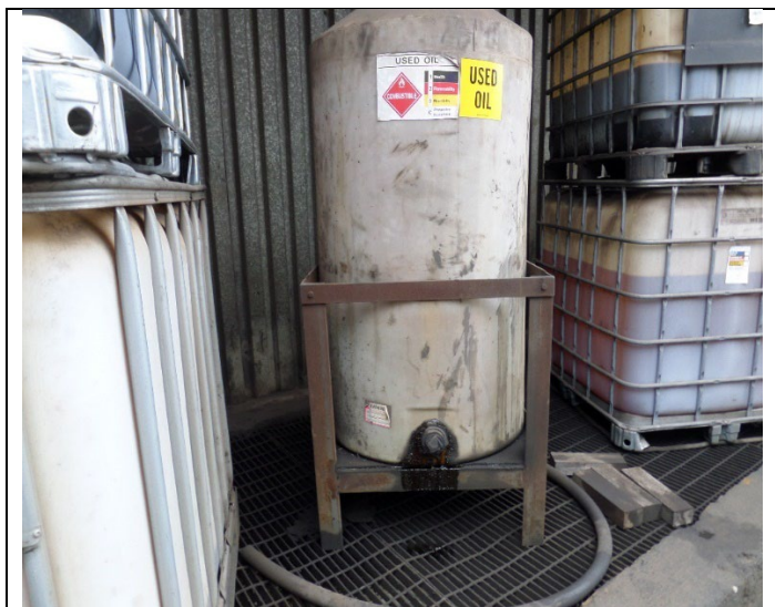
Cold Finishing Building - Used Oil Storage. Observed used oil on the bottom of 100-gallon container, the stand and around the valve. Photograph 19 taken at 1:46 p.m.
