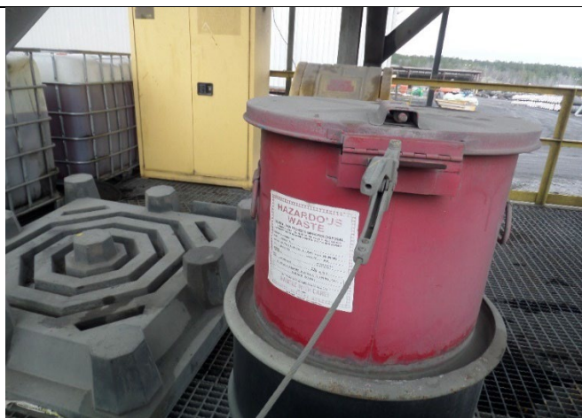
Used Oil Storage Area. Observed a 35-gallon SAA container. Photograph 6 taken at 11:18 a.m.
