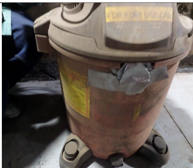
Baghouse #2 Basement SAA. Observed Nucor representatives closed the vacuum. Photograph 4 taken at 10:59 a.m.
