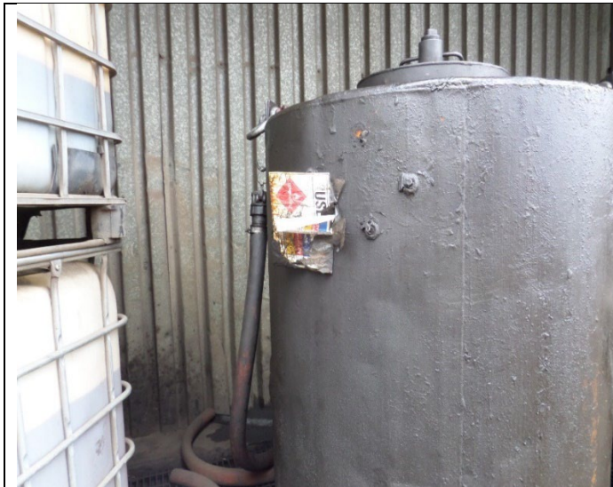
Cold Finishing Building - Used Oil Storage. Observed 300-gallon used oil container not marked or labeled clearly with the words used oil. Photograph 15 taken at 1:42 p.m.
