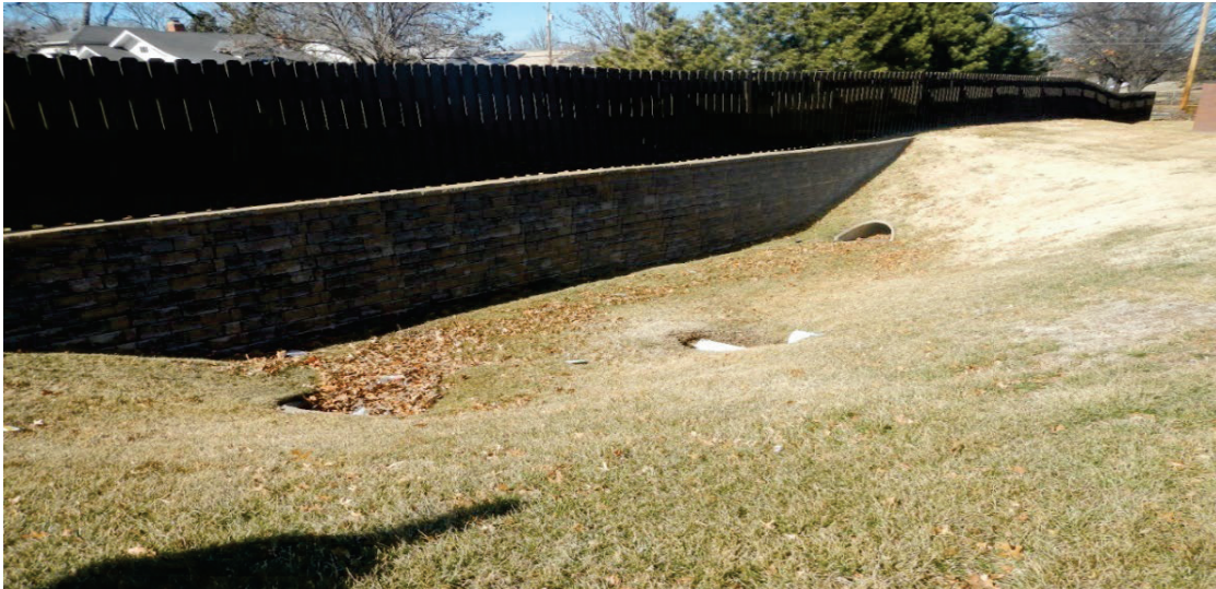
Photo 4, Dry detention basin at QuikTrip as a post-construction BMP.
