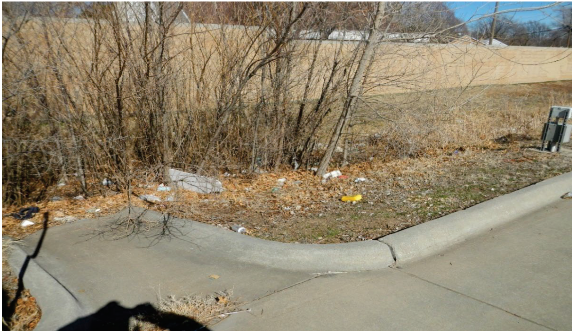
Photo 6, Dry detention basin at the Old Walmart as a post-construction BMP.
