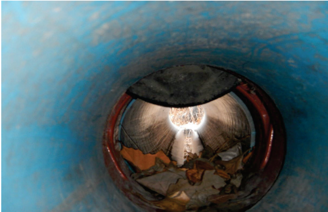
Photo 25, The north containment full of petroleum residue with an open valve
