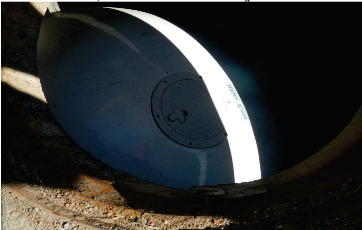
Photo 14, 72-inch Snout. Wichita's MS4 largest snout
