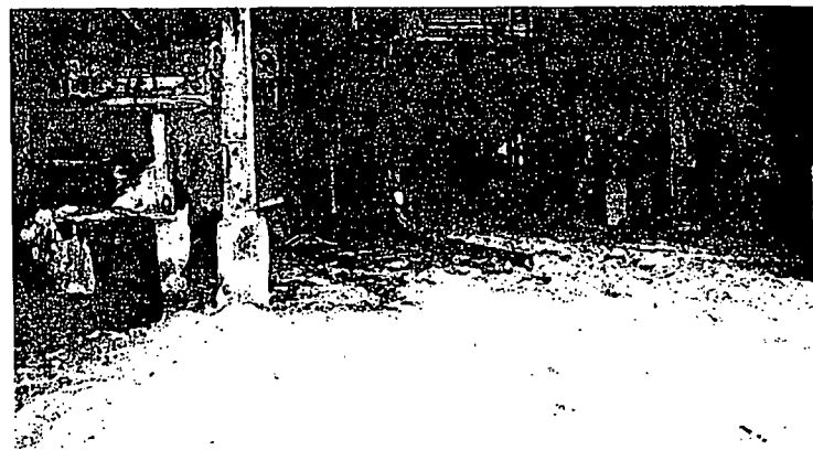
Gross contamination of friable asbestos coated every surface in the warehouse, often to a depth of several inches.
