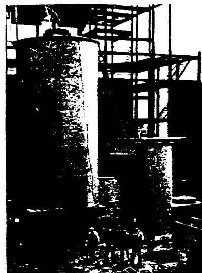
The impure hot sulphur dioxide gas enters the lead lined scrub tower, shown above, where it is cooled and partly purified.
