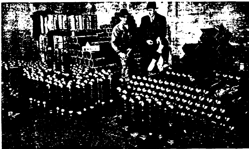
Plumbing foreman and the mechanical engineer inspecting the spun closed lead stubs before installation.
