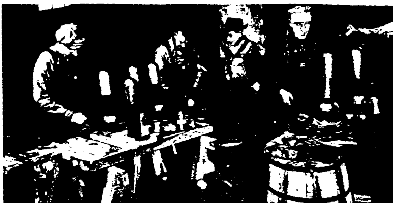
Plumbers at the lead bench preparing lead stubs for installation in the Terrace Plaza Hotel and Stores Building, Cincinnati, Ohio.
