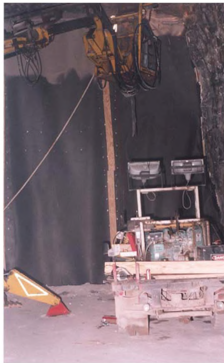
Figure 8. Fabric-grid material sprayed with cementitious material.
