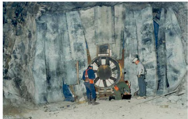
Figure 4. Used mine belt used pressure relief.
